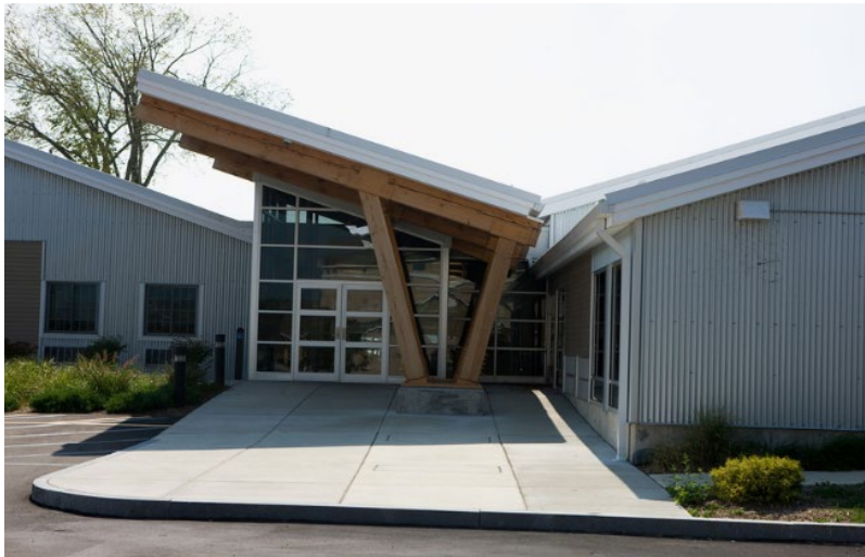
Figure 4. Statler Food Commissary Building (RTK Station Location)
