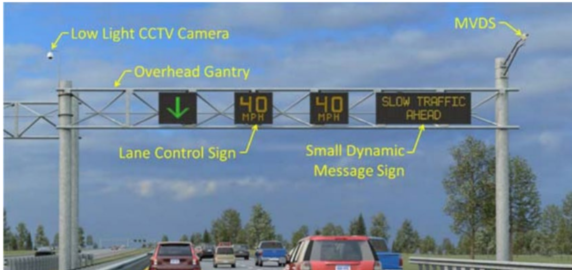
Figure 4 MDOT US23 FlexRoute Gantry
