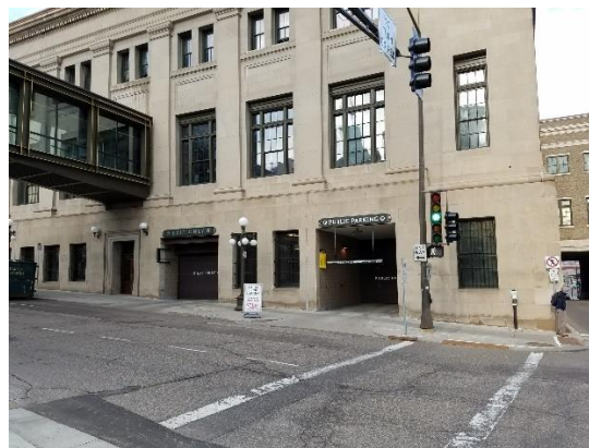
Figure 3.11: Parking Garage Entrance/Exit Close to an Intersection (source: Union Depot )
