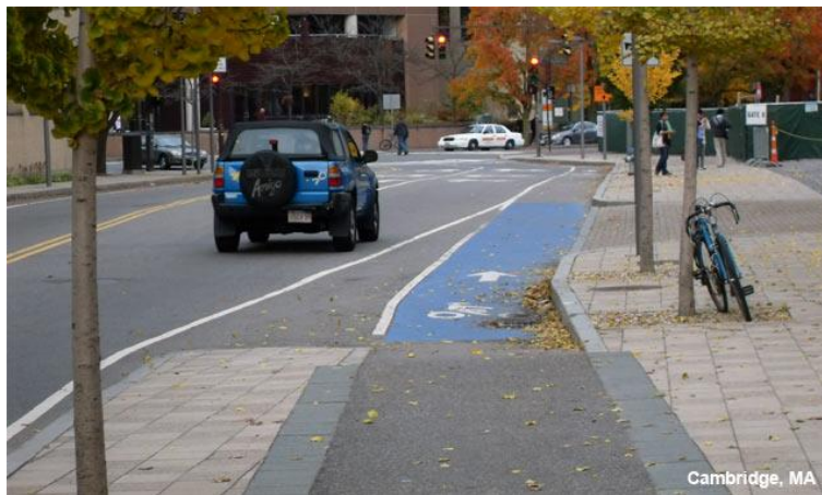
Figure 2.16: Cycle Track Intersection Approach (source: NACTO )
