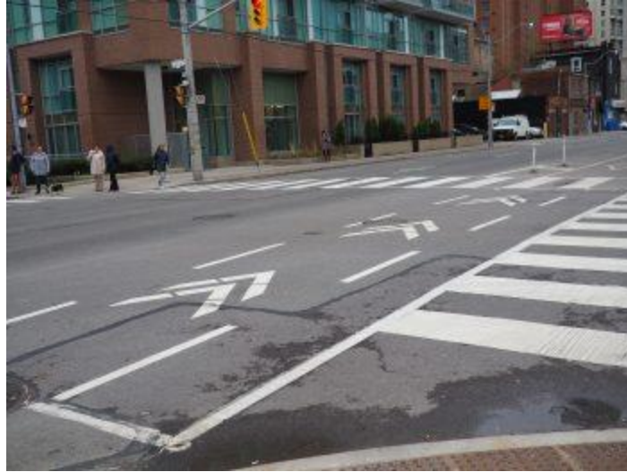
Figure 2.21: Intersection Crossing Marking with Dotted Lines and Chevrons (source: City of Toronto )
