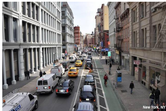
Cycle Track Separated with On-Street Parking
