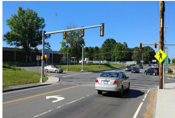
Signalized Intersection (source: Bayside Engineering )
