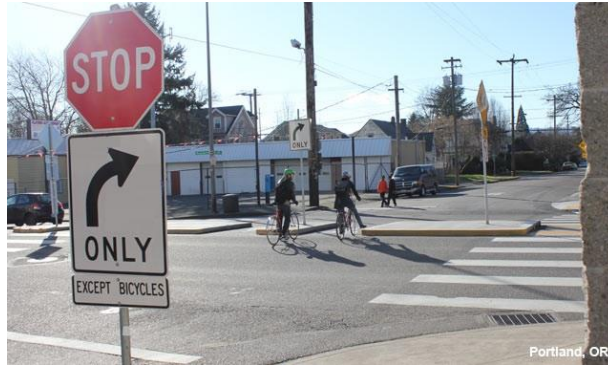
Figure 2.13: Median Refuge Island (source: NACTO)
