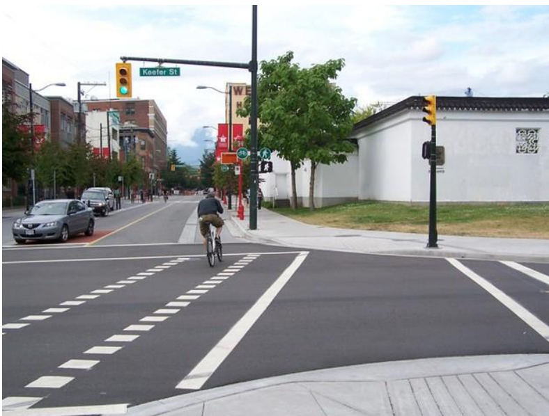
Figure 2.18: Intersection Crossing Marking with Elephant Feet (source: Flickr )
