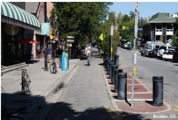
Cycle Track Separated with Boulders
