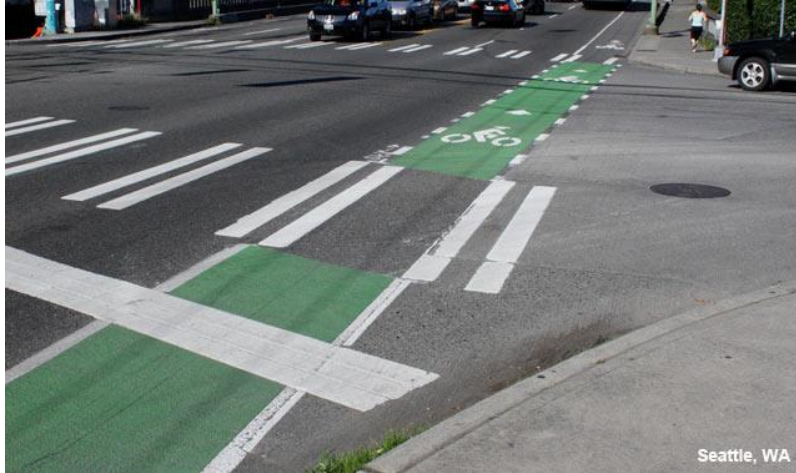
Figure 2.19: Intersection Crossing Marking with Dotted Lines and Colored Conflict Area (source: NACTO )
