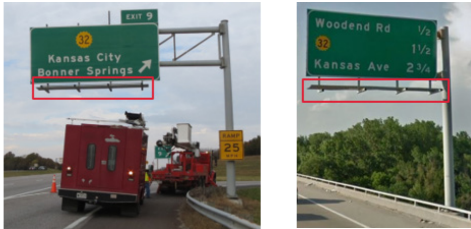
Figure 1.3: Examples of a steel grate walkway on a two-chord COSS
