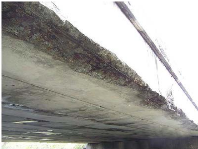
Figure 3.15 - Element 104: Box Girder, Prestressed Concrete CS-3
