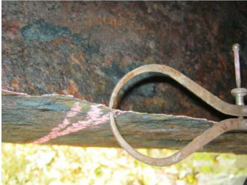
Figure 3.14- Element 107: Girder, Steel CS-4
