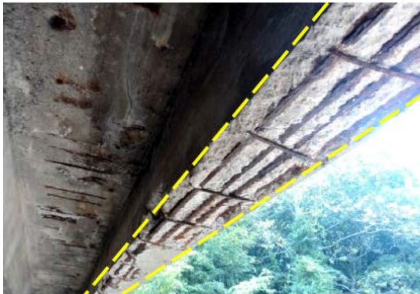
Figure 3.17 - Element 110: T-Beam, Reinforced Concrete CS-3
