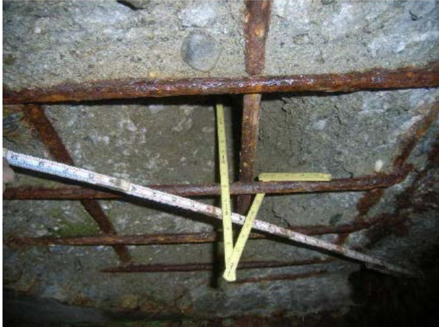
Figure 3.12 - Element 12: Reinforced Concrete Deck CS-4.
