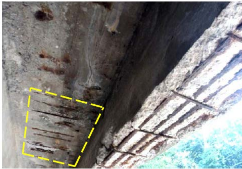
Figure 3.11 - Element 12: Reinforced Concrete Deck CS-3.
