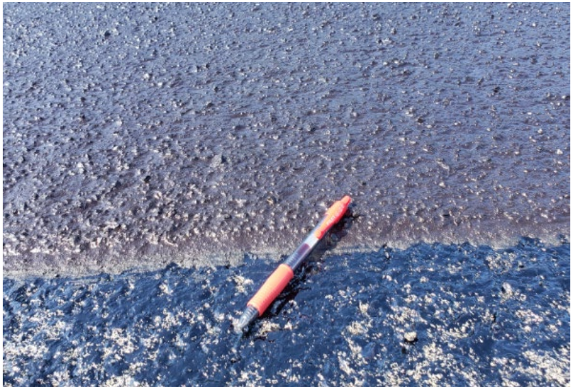
Microsurfacing slurry as it is setting on tack coated pavement
