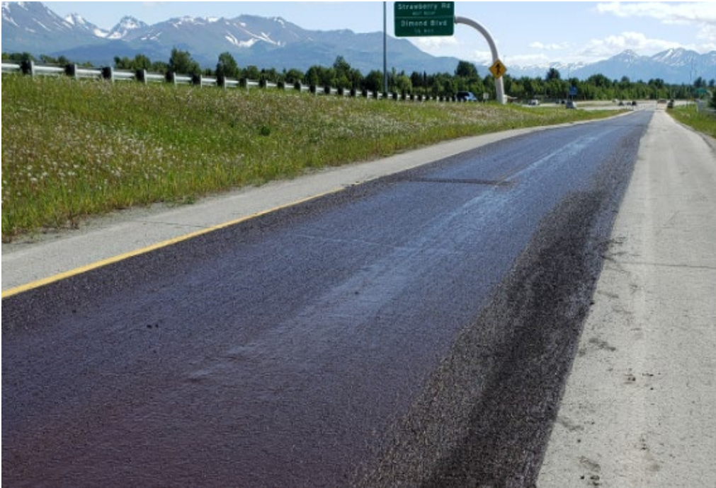
A hand worked area on the right side of the ramp on the scratch course on Ramp 11.
