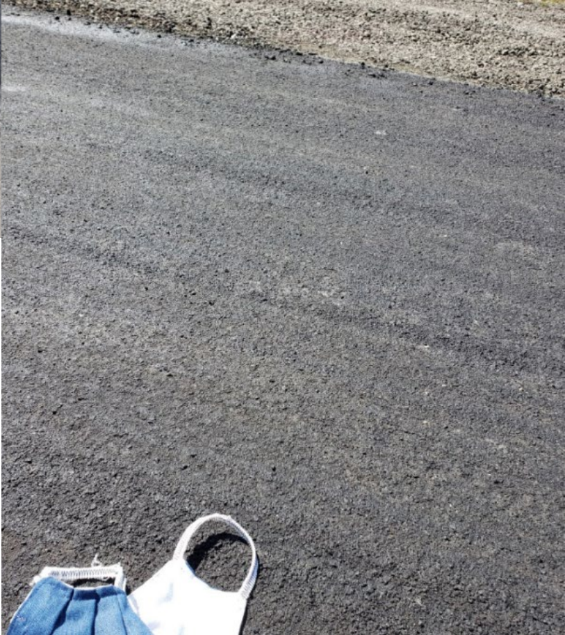
A mask on the microsurfacing test strip after the roller has made its passes and it has set.
