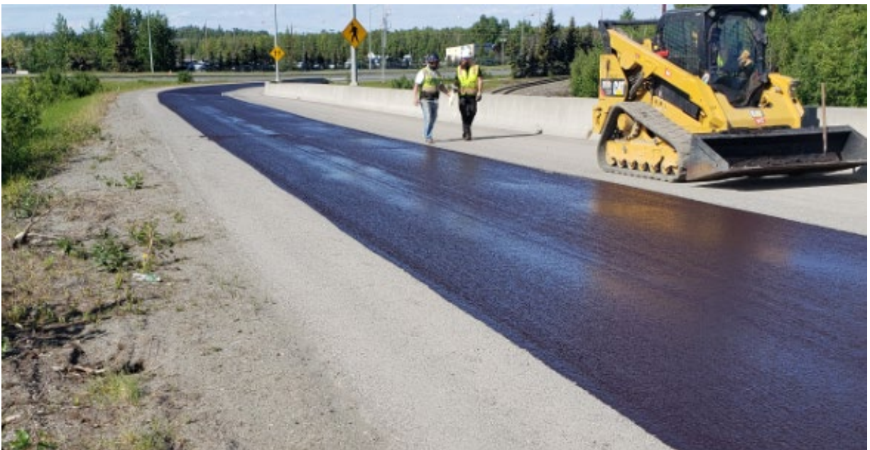
Scratch course placed on Ramp 5 prior to stopping production.
