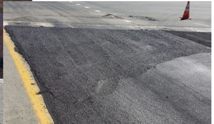
Photo 11 - Hand Worked Area on Ramp 6
