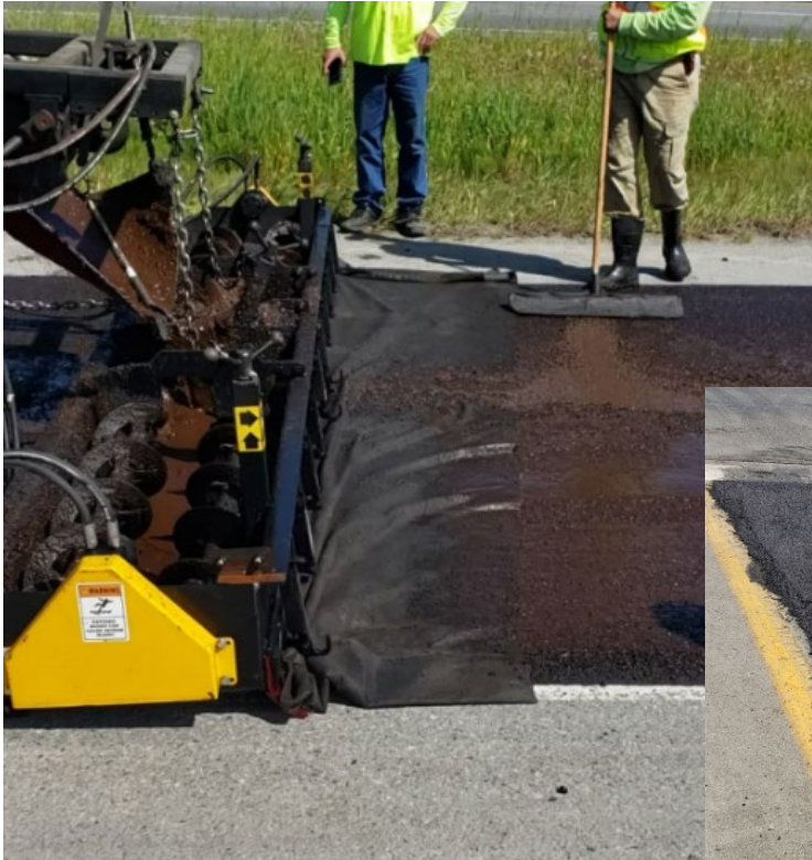
Photo 10 - Secondary Strike Off and Hand Working
