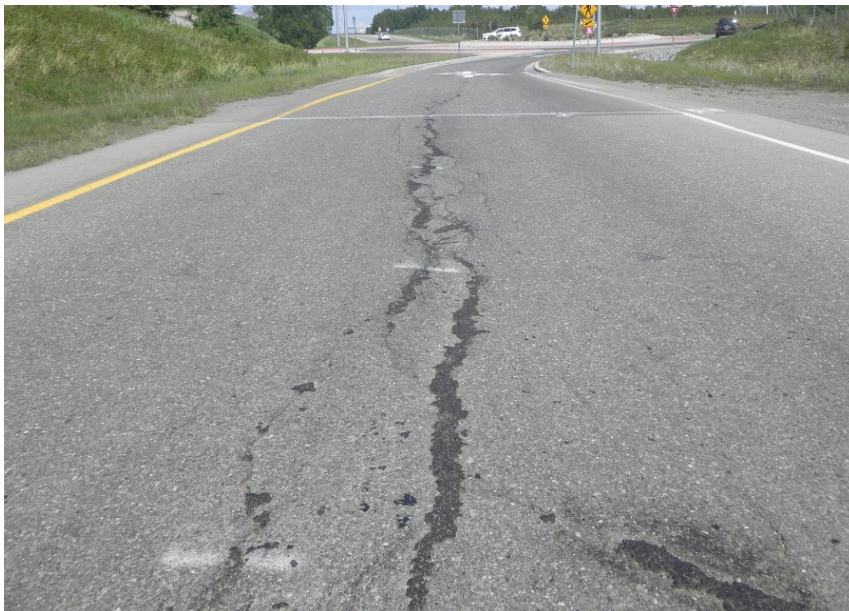
Photo 8 - Ramp 16 After Surface Preparation
