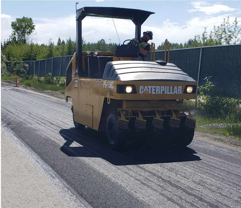
Photo 12 - Pneumatic Roller on Test Strip
