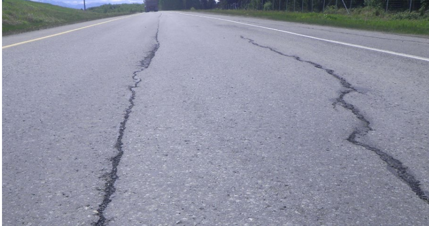
Photo 7 - Ramp 15 After Surface Preparation
