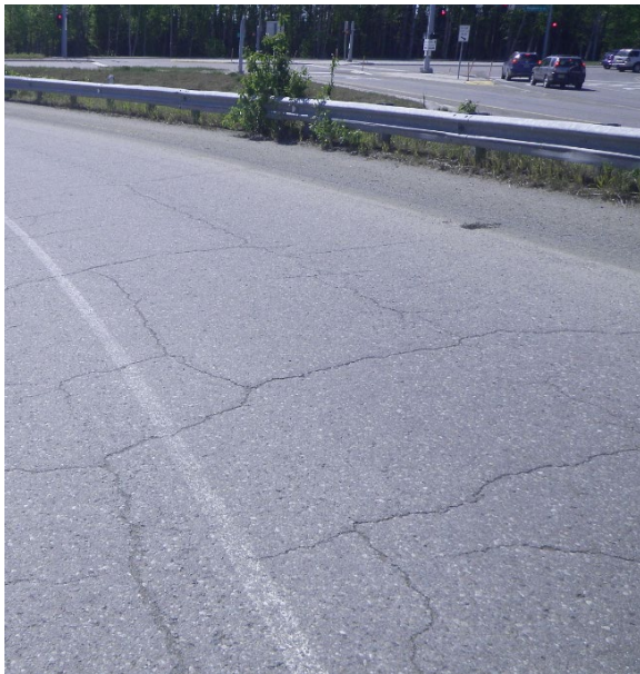
Photo 3 - Ramp 8 General Condition
