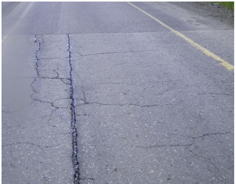
Photo 4 - Ramp 9 General Condition
