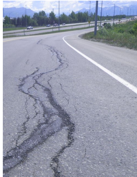
Photo 2 – Ramp 1 After Surface Preparation
