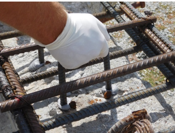
(e) Installing U-Shaped Bars
