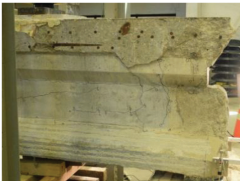
Figure 5.14 NSM FRP specimen prior to testing.
