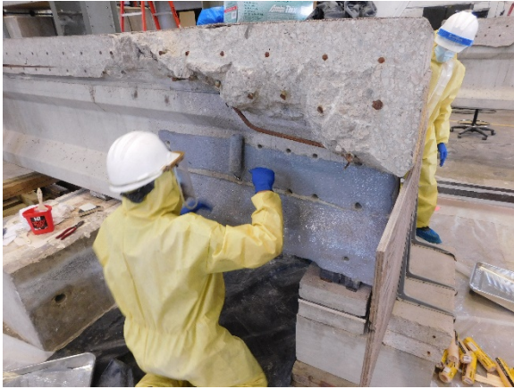
(a) Sealing Concrete Surface
