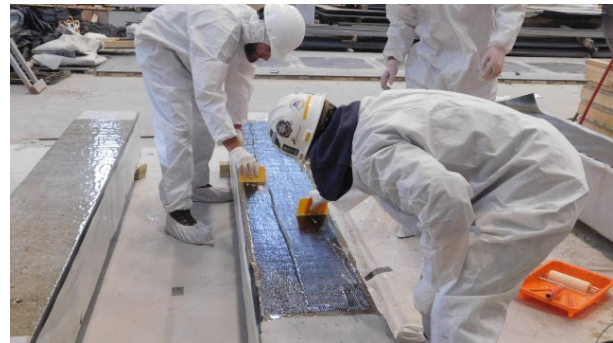
(f) Removing Excess Epoxy with Squeegee
