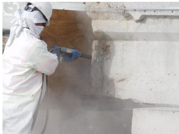
(b) Sandblasting to Remove Corrosion
