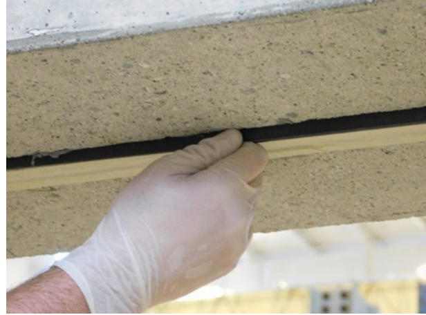
(b) Inserting NSM Strip
