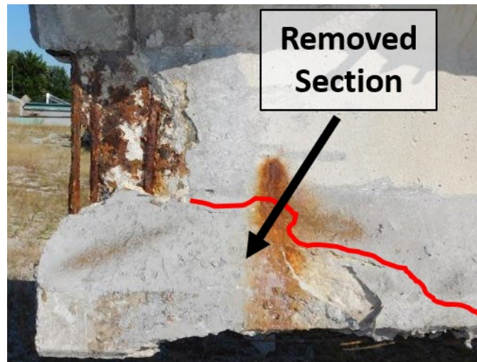
Figure E.18 Flange portion removed from supplemental diaphragm specimen.
