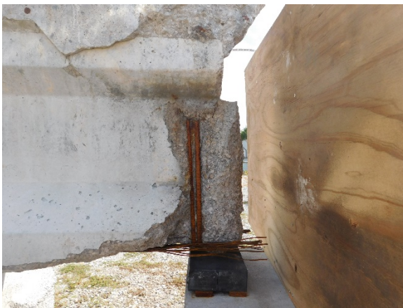
(c) Condition After Sandblasting
