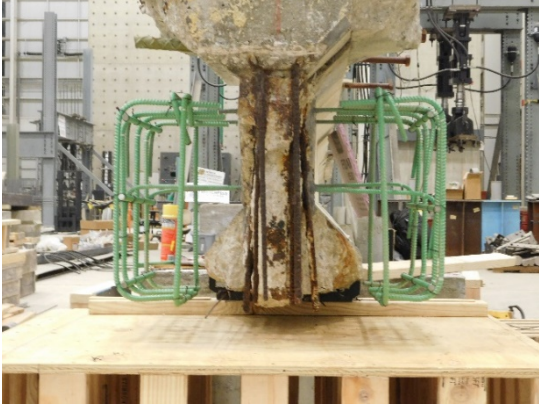
(k) Completed Reinforcing Cage
