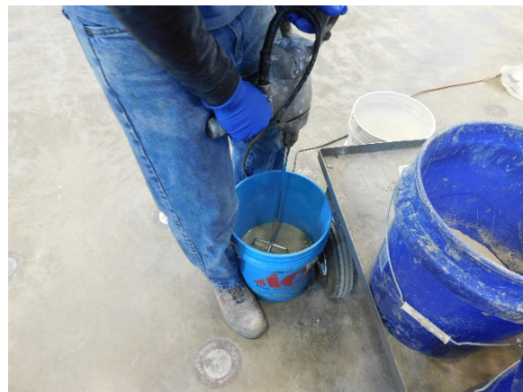
(b) Mixing Mortar
