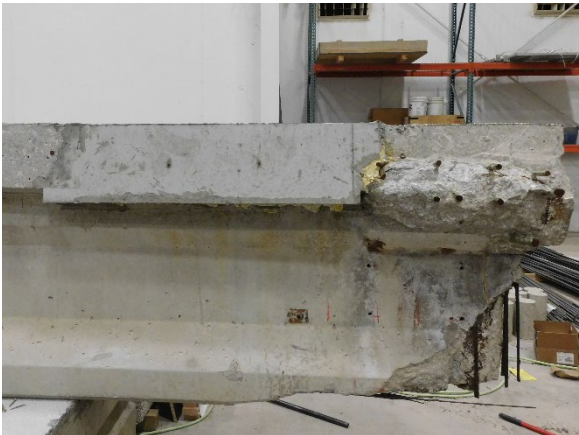
(c) Completed Deck Repair
