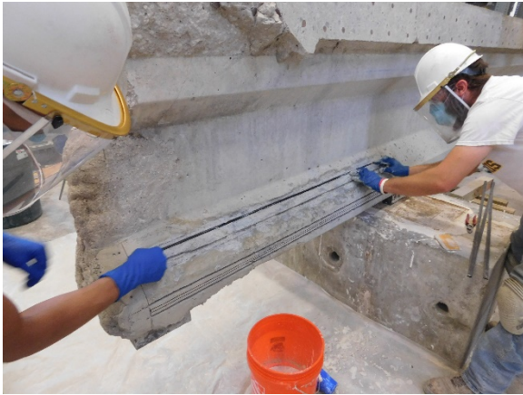
(c) Inserting NSM Strip
