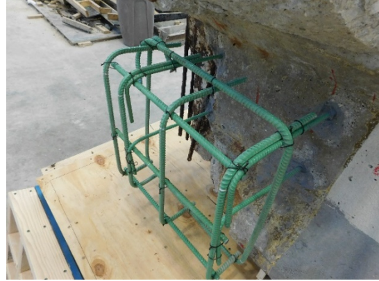
(l) Completed Reinforcing Cage
