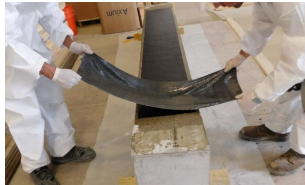
(b) Placing U-Wrap Anchor
