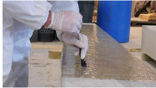
(b) Coating Inside of Drilled Holes with Epoxy
