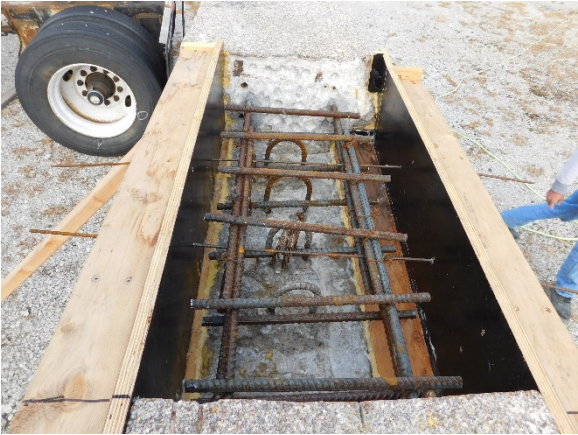
(a) Erected Formwork
