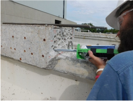
(a) Dispensing Epoxy for Anchorage of Longitudinal Reinforcement
