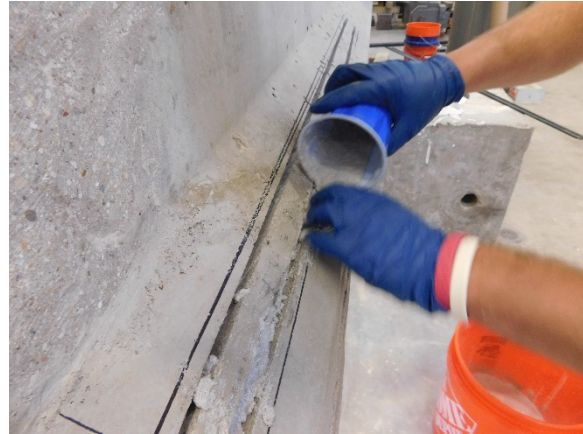
(b) Filling Groove with Epoxy Grout
