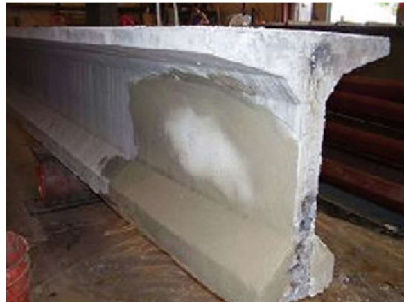
(b) Cross Section Restored
