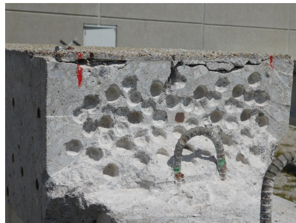
(d) Roughened Surface at End of Repair Area
