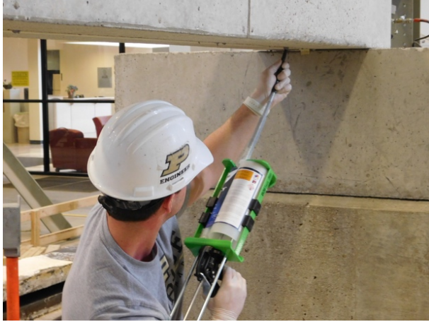
(a) Filling Groove with Epoxy
