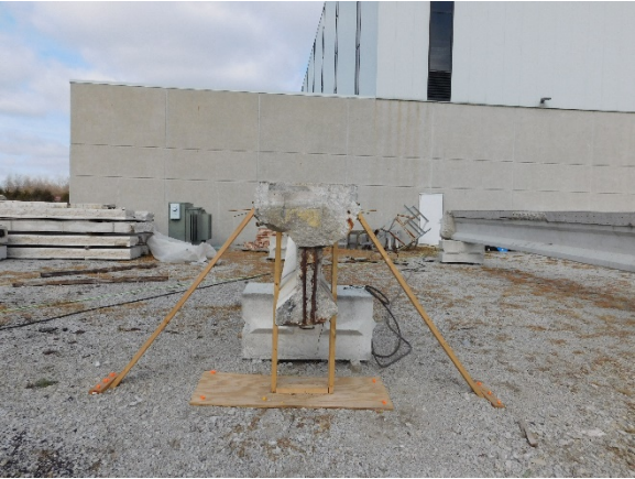
(b) Formwork Supports
