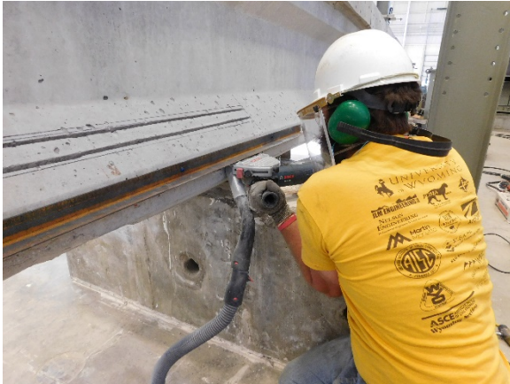
(a) Cutting NSM Groove
