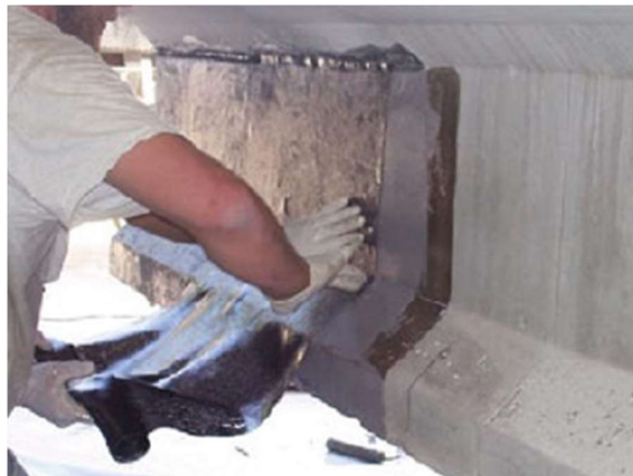
(f) FRP Repair
