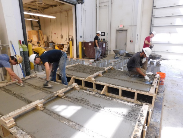
(b) Finishing Concrete
