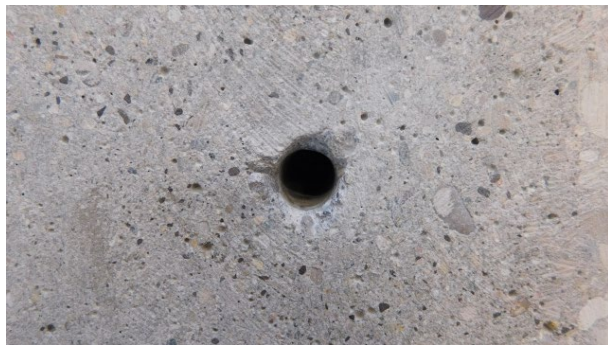
(c) Drilled Anchor Hole Prior to Rounding Edges
