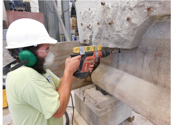
(f) Drilling Anchor Holes
