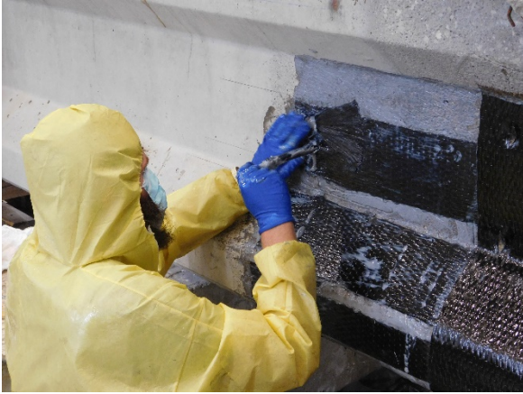
(c) Inserting Spike Anchor
