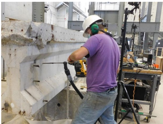
(a) Drilling Holes for No. 3 Bars
