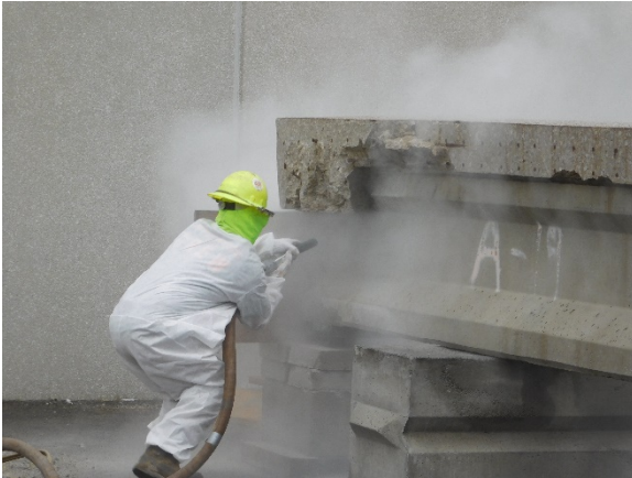
(e) Sandblasting for FRP Application
