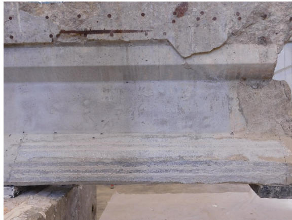
(e) Completed NSM Repair System
