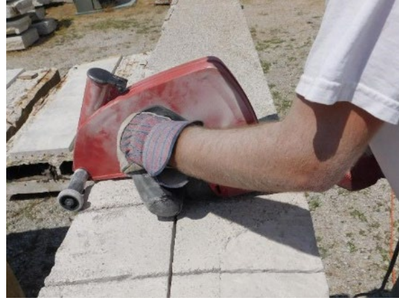
(b) Sawing Concrete Deck
