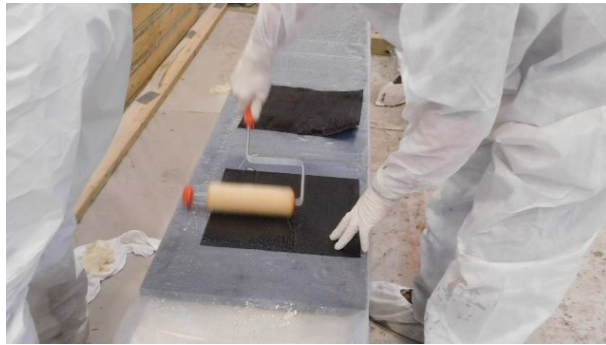
(a) Saturating Patch Sheets
