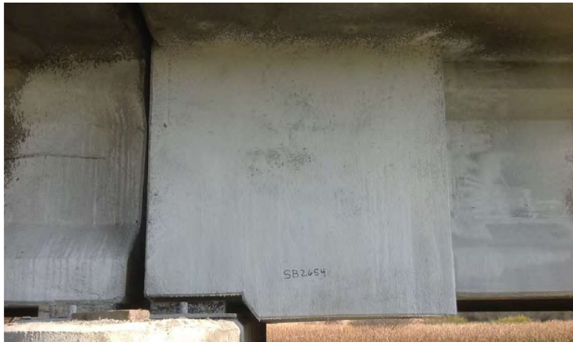
(b) Complete Shotcrete Repair
