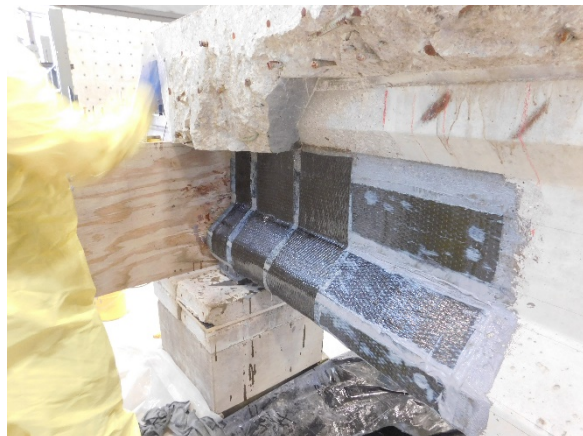
(f) Externally Bonded Strips/Sheets Applied to Specimen
