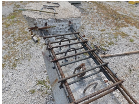
(f) Completed Reinforcement
