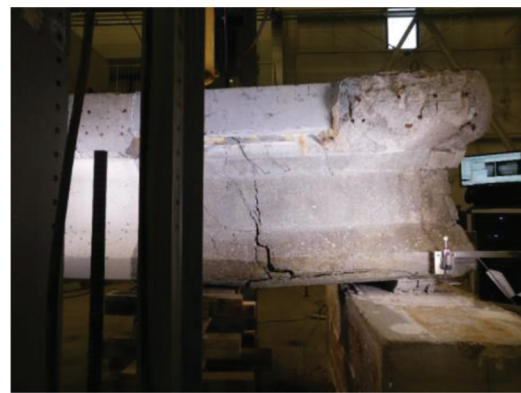
Figure 4.7 Damaged specimen after failure.
