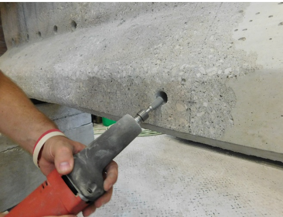
(g) Rounding Edges of Anchor Hole
