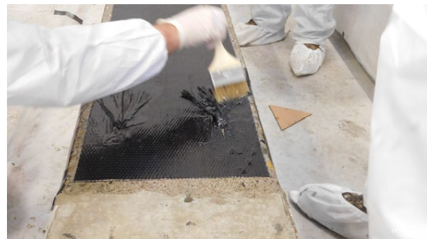
(f) Saturating Anchors
