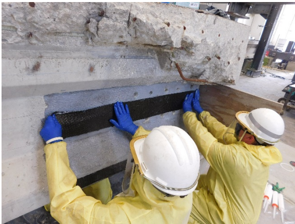
(c) Placing Longitudinal Strips
