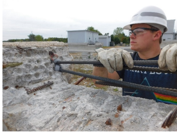
(b) Inserting Longitudinal Reinforcement
