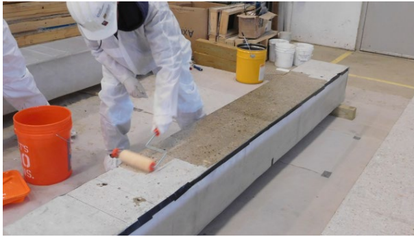
(a) Sealing Concrete Surface
