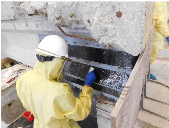
(e) Removing Excess Epoxy with Squeegee
