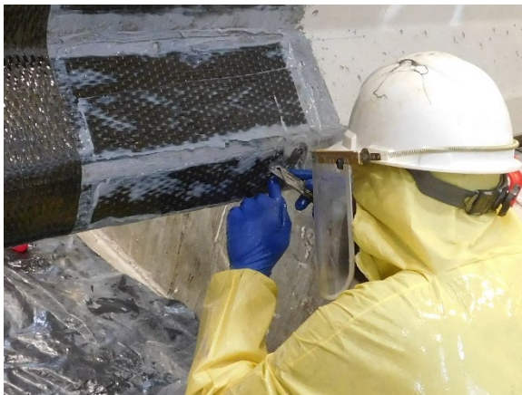
(a) Separating Fibers with Razor Blade
