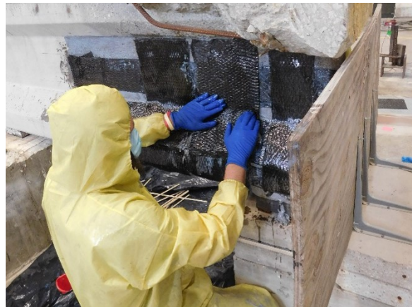
(h) Placing Patch Sheets
