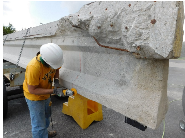
(h) Rounding Girder Edges
