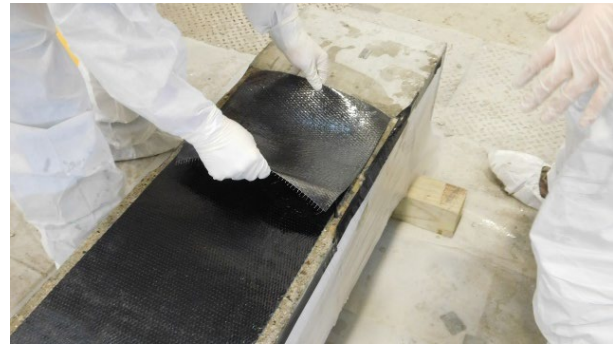
(b) Placing Patch Sheets
