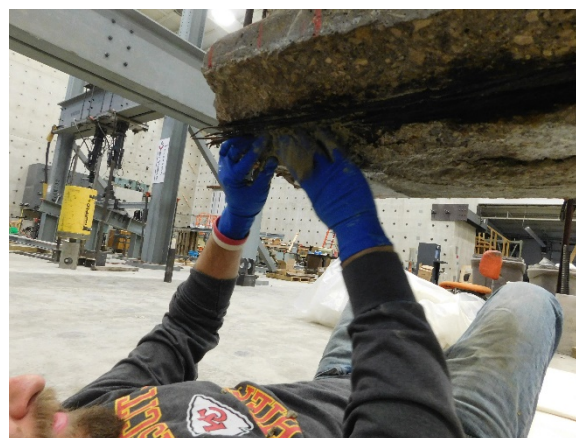
(c) Placing Mortar
