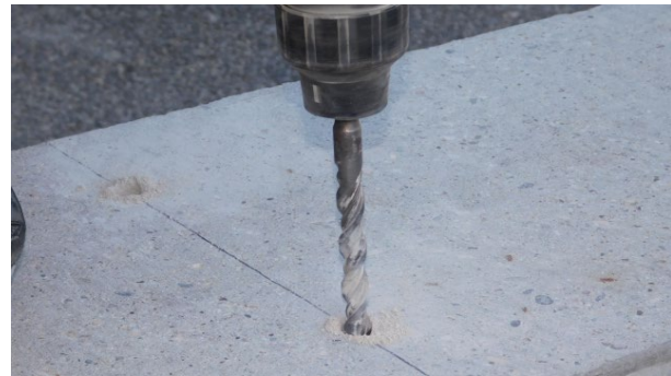
(b) Drilling Anchor Holes
