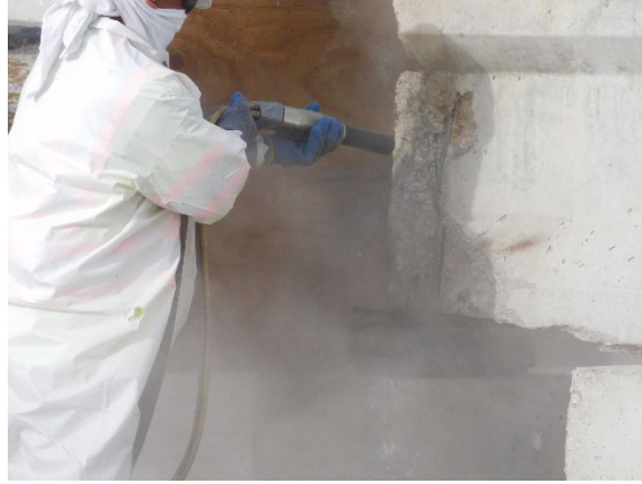
(b) Sandblasting to Remove Corrosion
