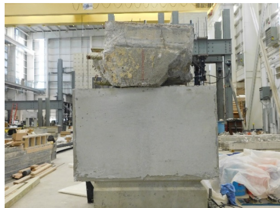
(p) Completed Supplemental Diaphragm Repair System
