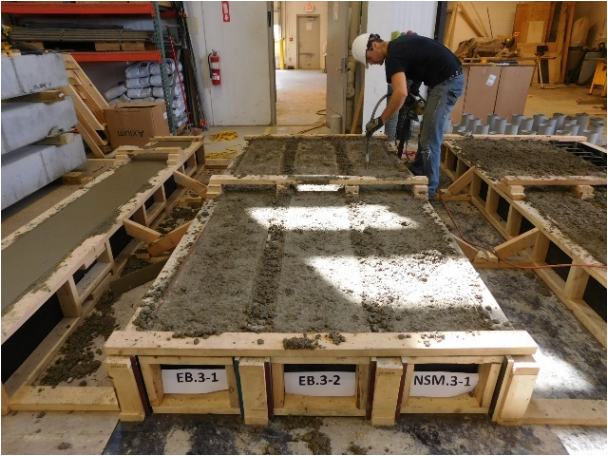
(a) Vibrating Concrete into Place
