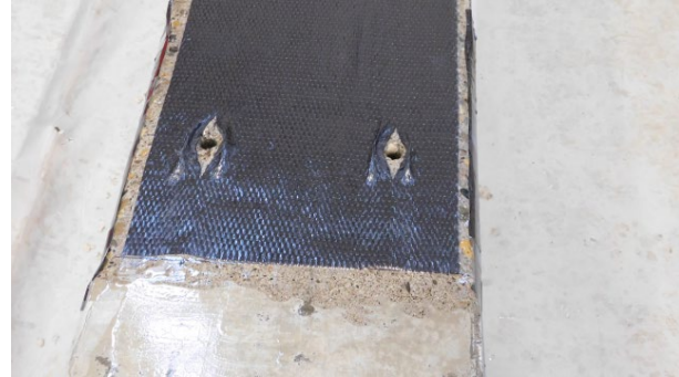
(b) Exposed Anchor Holes
