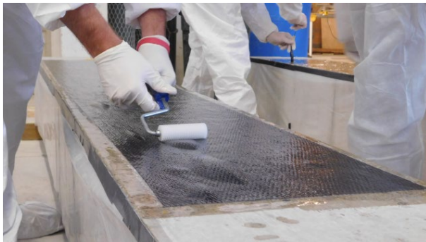
(e) Rolling FRP Sheet to Eliminate Air Pockets
