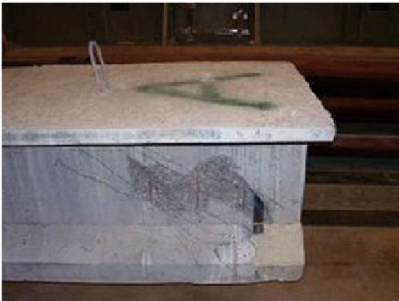
(a) Delaminated Concrete Removed
