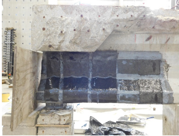
(i) Completed Externally Bonded FRP Repair System
