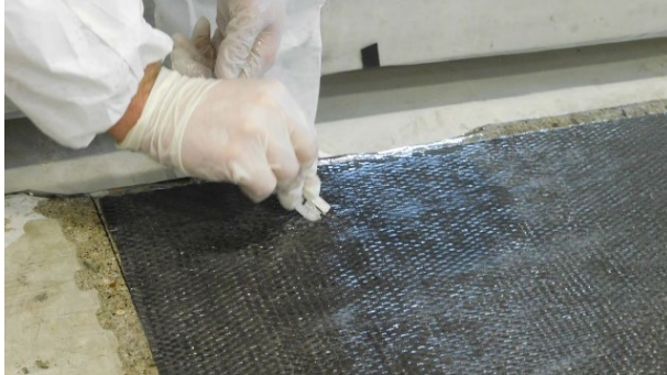
(a) Separating Fibers with Razor Blade
