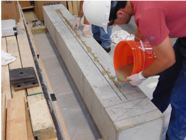
(a) Filling Groove with Epoxy Grout
