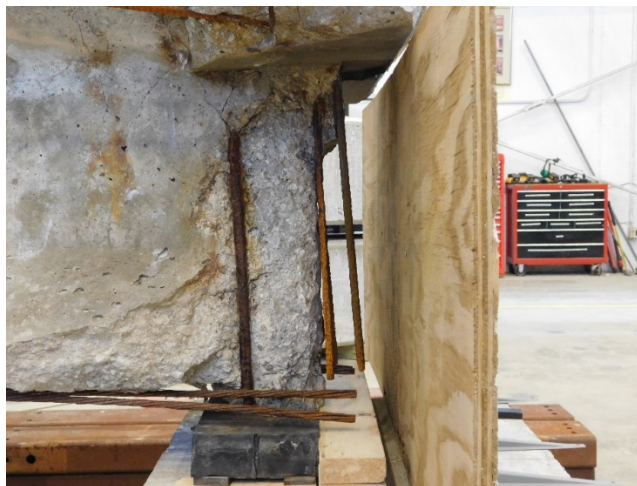
Figure E.9 Simulated mud wall and bearing pad location for externally bonded FRP specimen.
