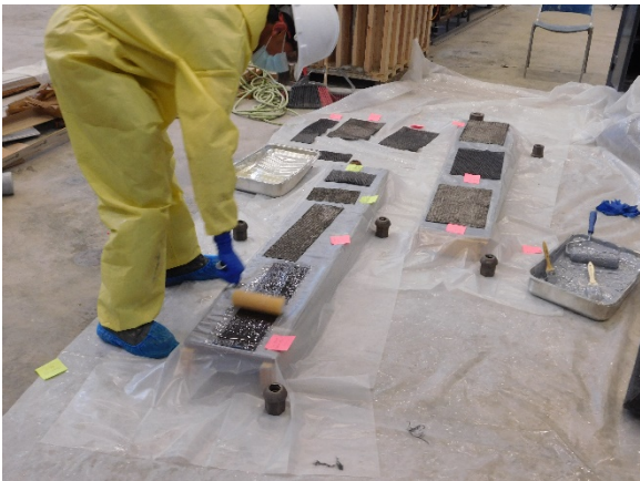
(g) Saturating Patch Sheets
