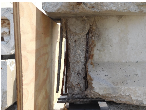
(c) Condition After Sandblasting
