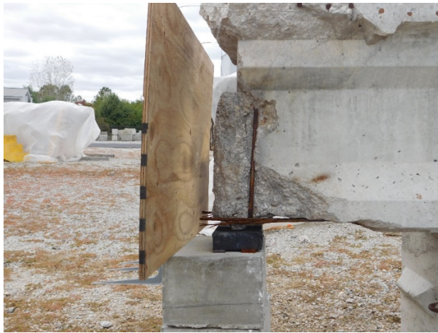
Figure E.15 Simulated mud wall and bearing pad location for NSM FRP specimen.
