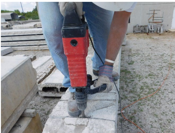
(c) Removing Concrete to Create Rectangular Repair Area
