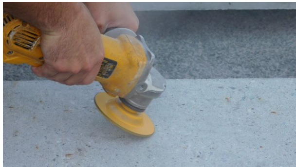
(a) Grinding Concrete Substrate
