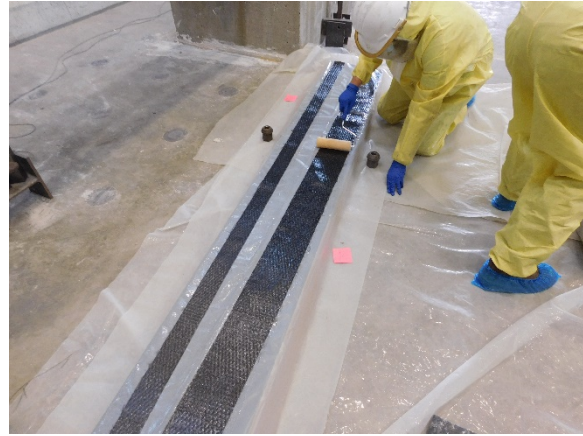
(b) Saturating Longitudinal FRP Strips
