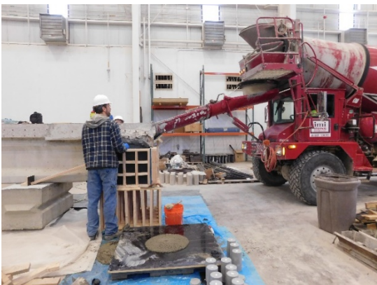
(o) Casting SCC
