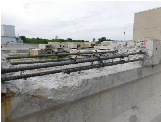
(c) Longitudinal Reinforcement After Placement
