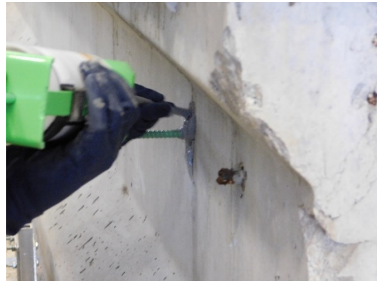
(h) Injecting Additional Epoxy
