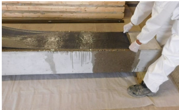
(a) Placing Longitudinal Sheet
