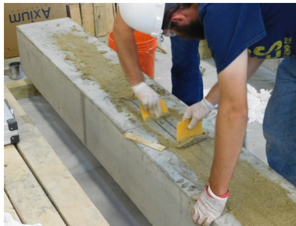
(c) Leveling Off Excess Epoxy Grout
