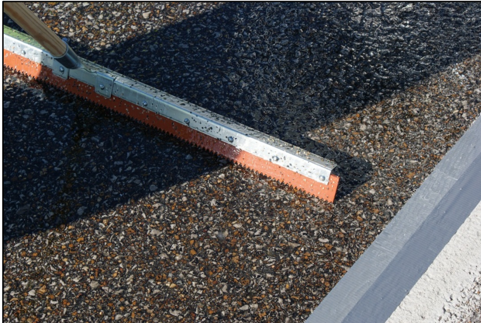
Figure 2.2. Example of notched squeegee used to distribute epoxy to pavement surface.
