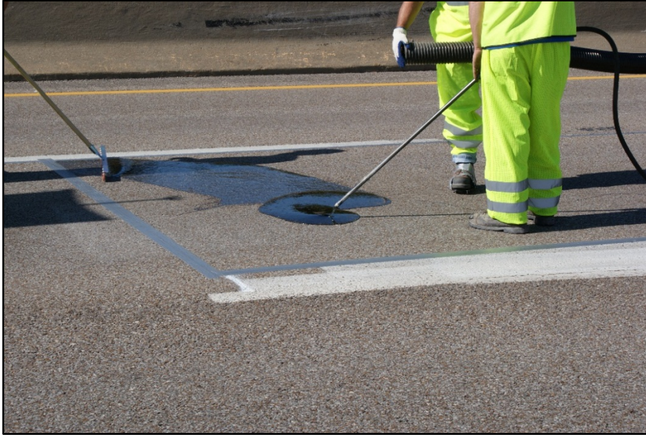
Figure 2.1. Example of application of epoxy to road surface using sprayer wand.
