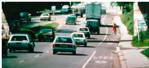
FIGURE 3: Designated on-street bicycle lane
