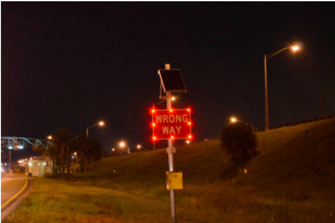
Figure 2-1 Example of LED-Enhanced Wrong-way Sign
