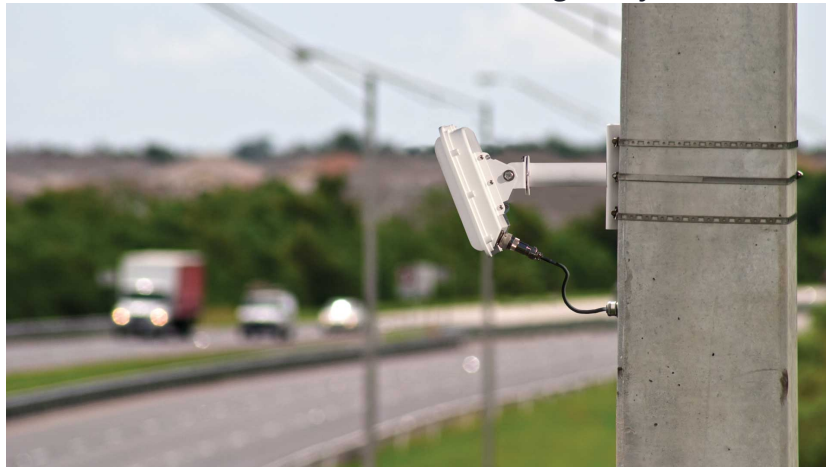
(b) Installation of Smartsensor HD on an existing pole
