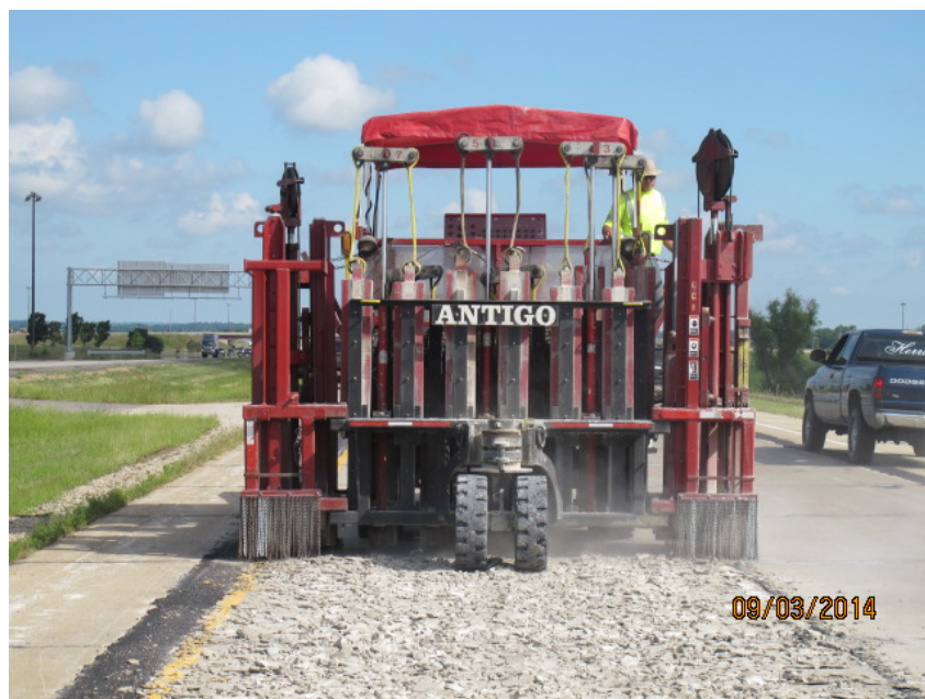
Figure 9. Photo. Version of multi-head breaker common on Illinois projects.
