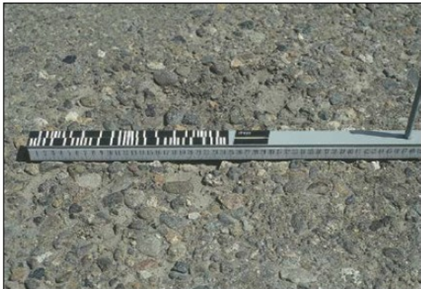
Loss of coarse aggregate
