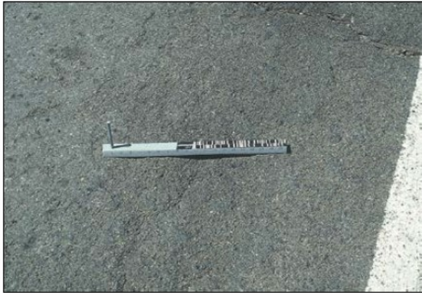
Loss of fine aggregate
