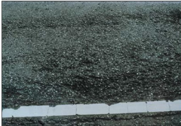
Loss of fine aggregate
