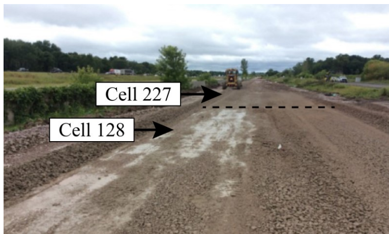
Figure 3.6. Subbase layers of Cells 128 and 227 (Van Deusen et al. 2018)
