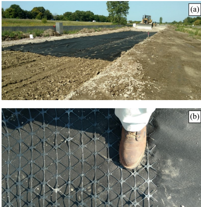
Figure 3.8. Placement of (a) geotextile and (b) triaxial geogrid over geotextile (White and Vennapusa 2017)
