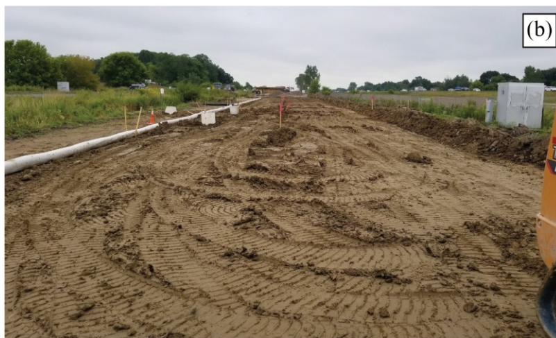
Figure 3.3. (a) Moisture content adjustment for subgrade soil and (b) prepared subgrade (White and Vennapusa 2017)
