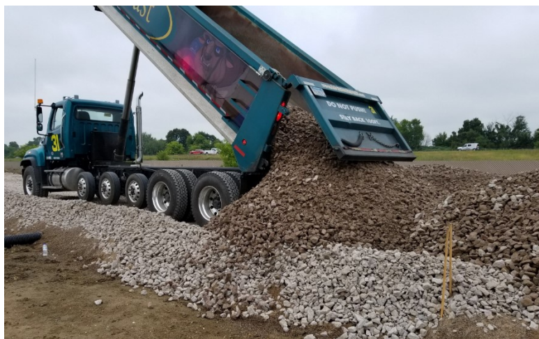
Figure 3.4. Placement of LSSB Material (White and Vennapusa 2017)
