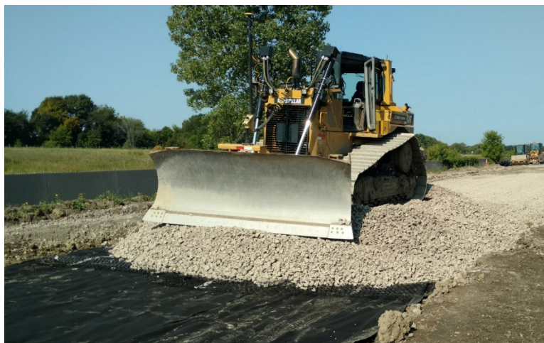
Figure 3.9. Placement of LSSB Material over geosynthetics (White and Vennapusa 2017)
