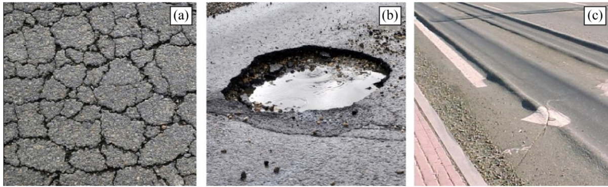
Figure 1.2. (a) Fatigue cracking [ https://texasmaterialsgroup.com/alligator-cracking-asphalt-repair/ (date accessed: January 23, 2021)], (b) pothole [ https://theconversation.com/potholes-how-engineers-are-working-to-fill-in-the-gaps-102055 (date accessed: January 23, 2021)], and (c) permanent deformation [ http://www.pavementinteractive.org/wp-content/uploads/2008/05/Mvc-037s.jpg (date accessed: January 23, 2021)]
