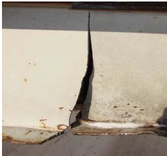
Cracking/Fatigue
