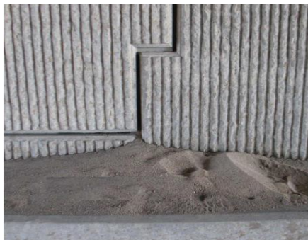
Loss of Backfill
