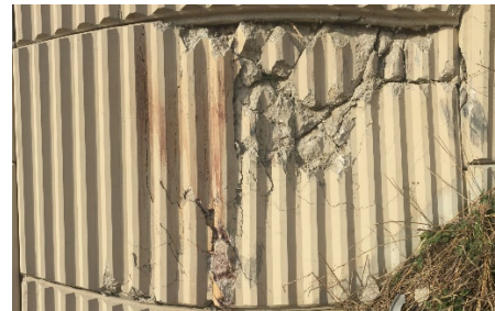
Deteriorated Panel
