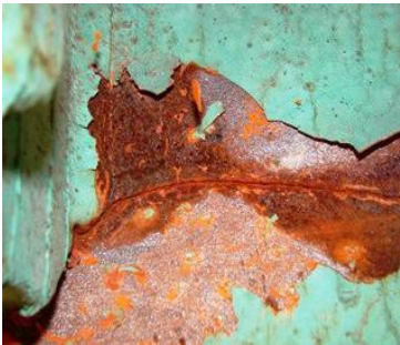
Cracking/Fatigue
