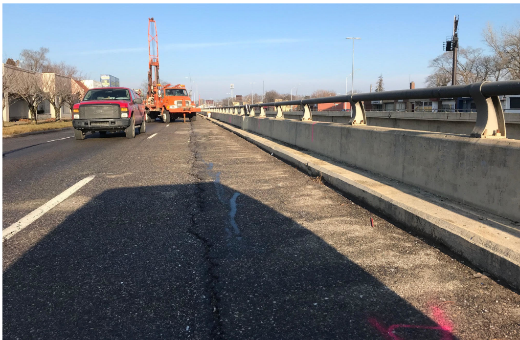
Figure B.2. Top road surface at the top of the suspected failed M-10 wall panel (January 2020); major tensile crack in asphalt surface evident parallel to wall face.
