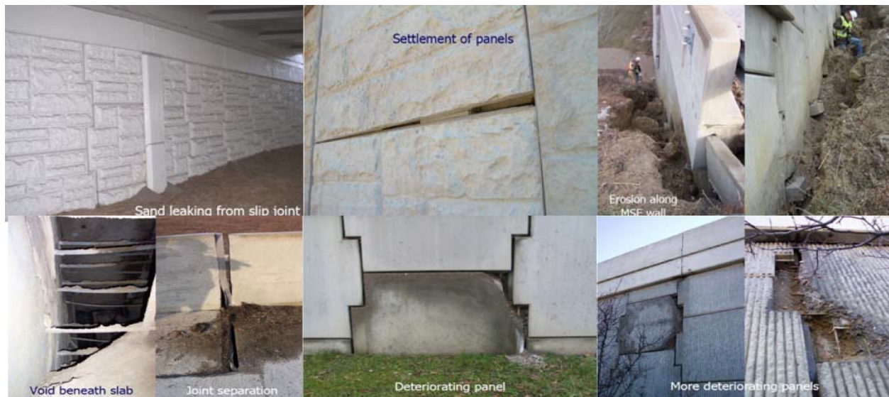
Figure 1.9. Observed problems in MSE walls (Narsavage 2006)
