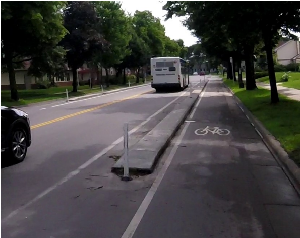
Buffer 3: Curb and Intermittent Barrier
