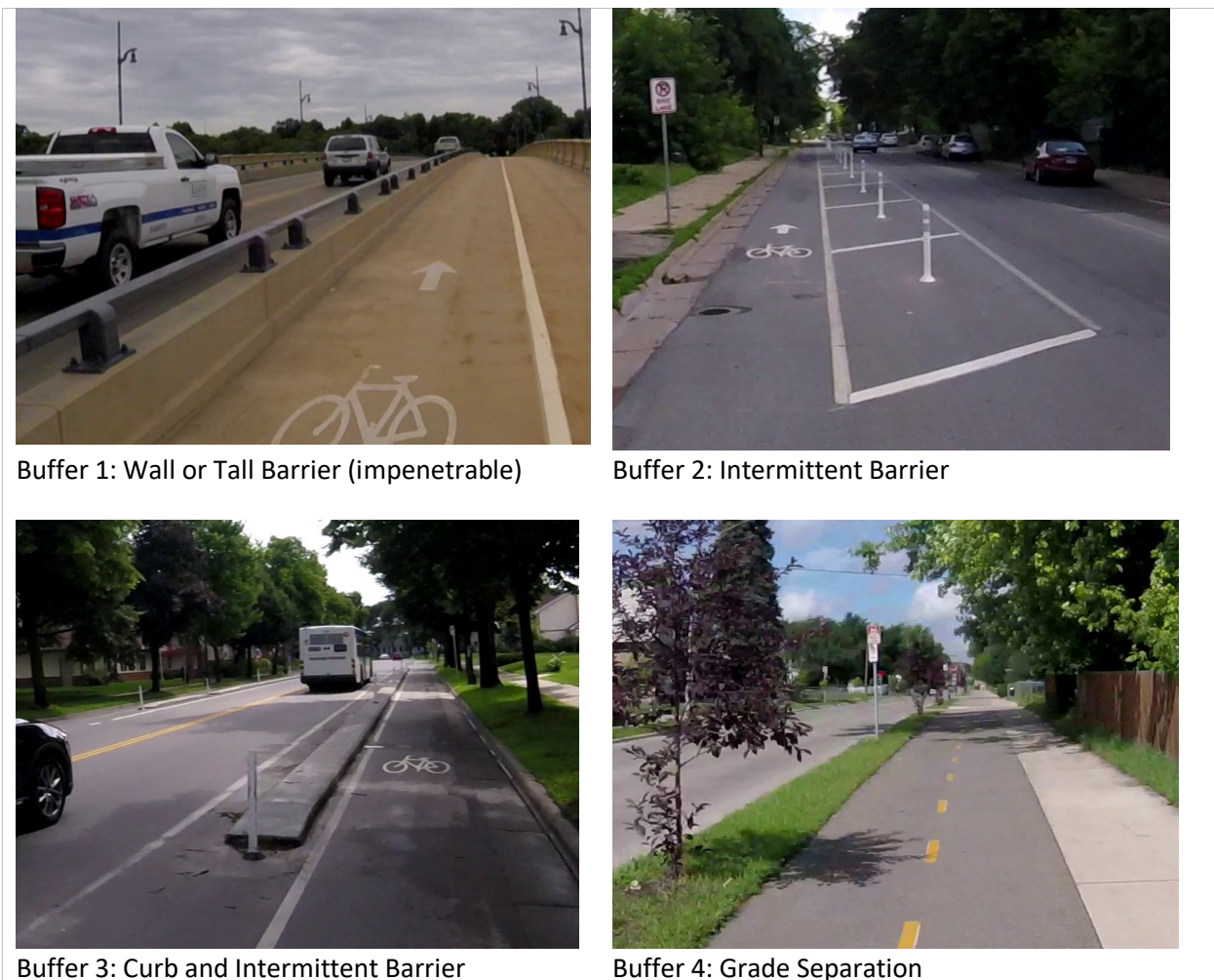
Figure 8.1 Types of Buffers Separation Methods
