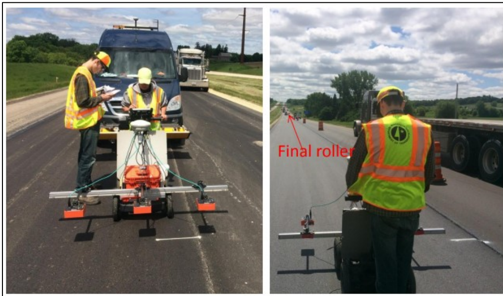
Figure 2.4: Equipment and Data Collection before a 500 ft pass (left), and during data collection moving behind the final roller compactor (right). (Hoegh & Dai, 2017)
