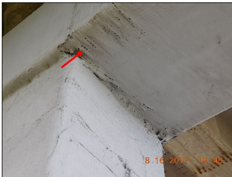
Figure B.135 Gaps between fiber tows within sheets.
