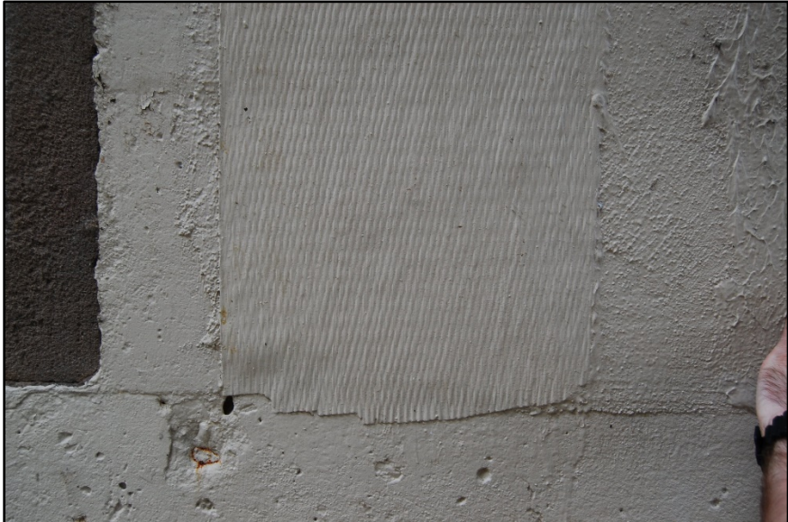
Figure B.11 Close-up of cut made to CFRP sheet.
