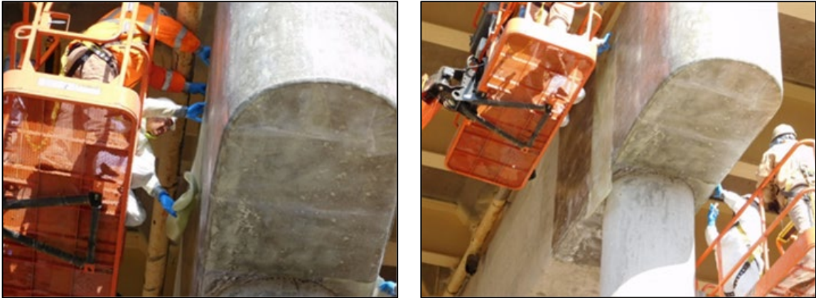
Figure B.189 Applying saturated FRP sheets to pier cap.
