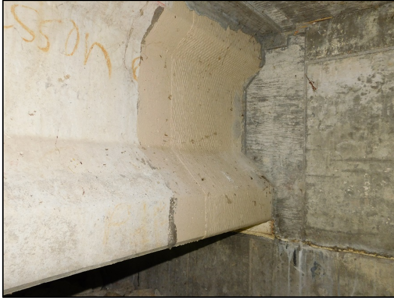
Figure B.56 Beam end repair at southern abutment.
