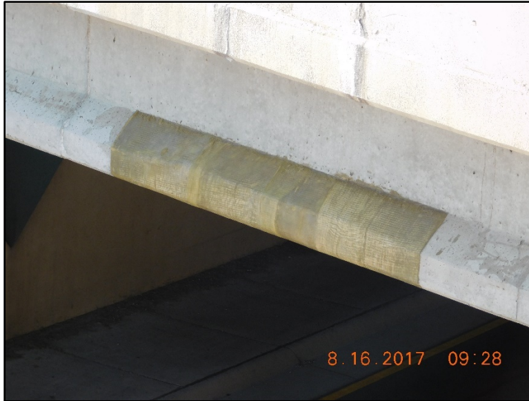
Figure B.104 Wrapping at impacted region.
