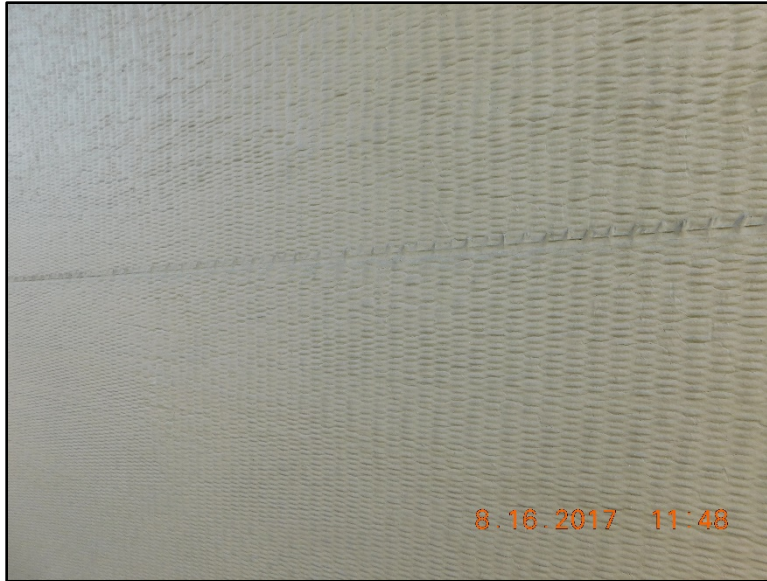
Figure B.118 Proper smooth surface of repair.
