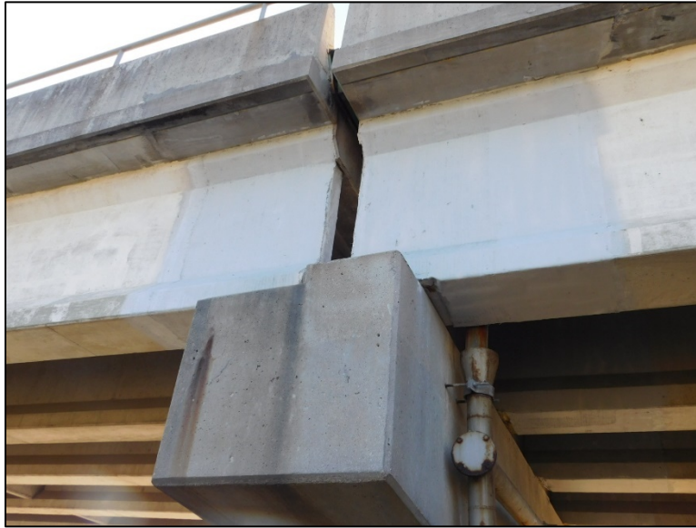
Figure B.163 Beam end repairs at joint near IN-156.
