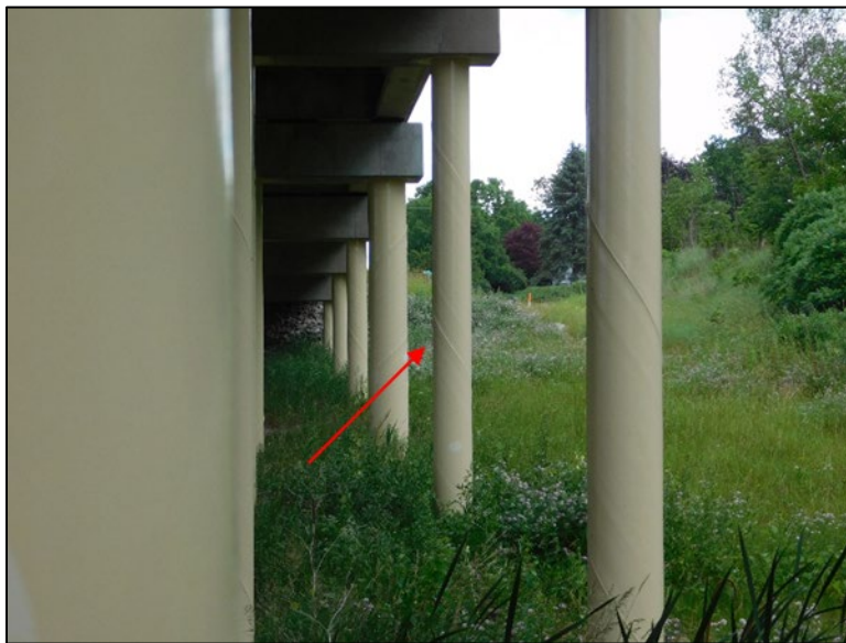
Figure B.57 Different column width from steel jacking.
