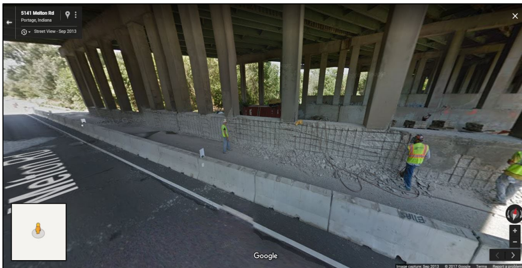
Figure B.19 Repair procedures on Bent 5, September 2013 (Google, 2013).
