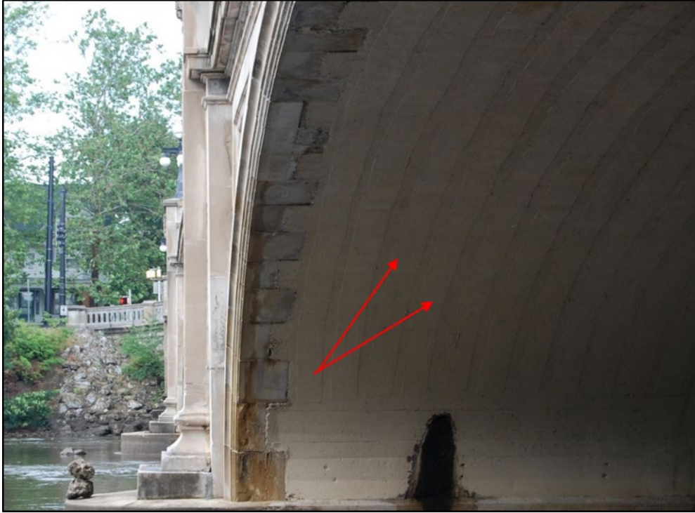
Figure B.10 CFRP strips on southern span.
