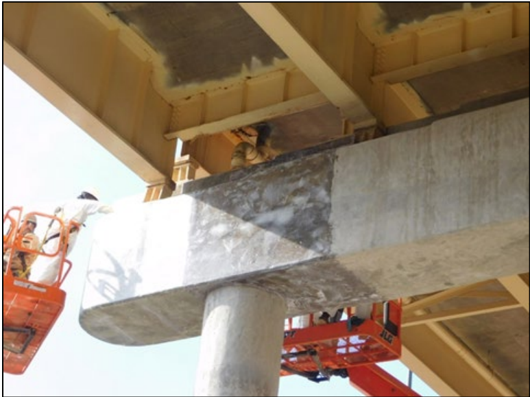
Figure B.188 Epoxy application to pier prior to FRP sheet application.
