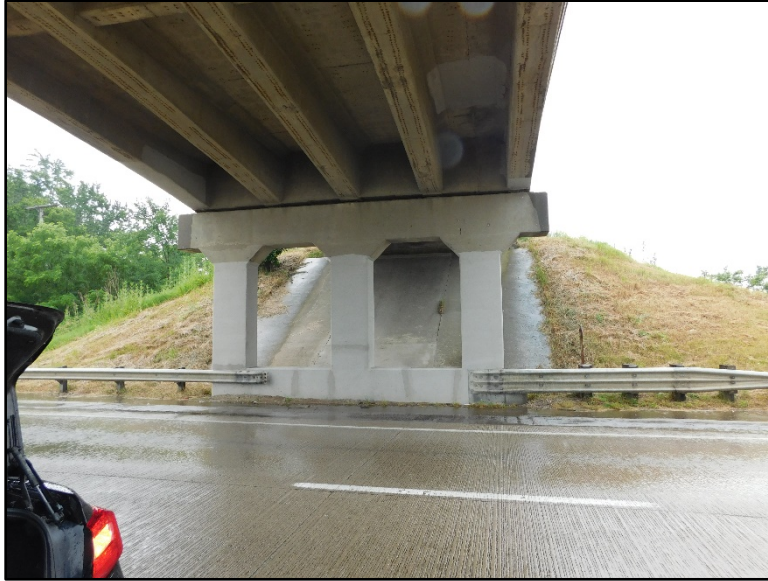
Figure B.33 View of the FRP-repaired western end pier.
