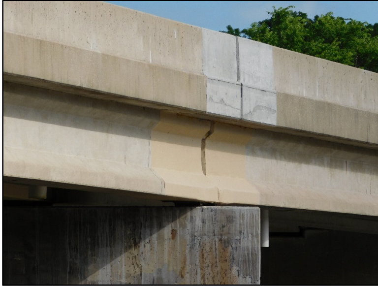
Figure B.72 Beam end repairs at southbound bridge Pier 4.
