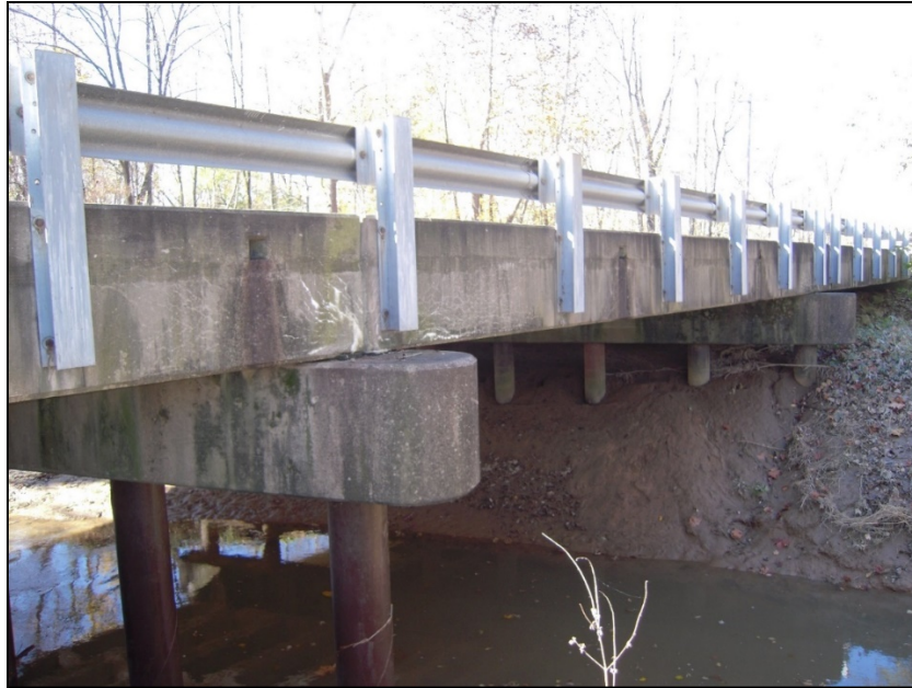
Figure B.146 Panoramic view of bridge.
