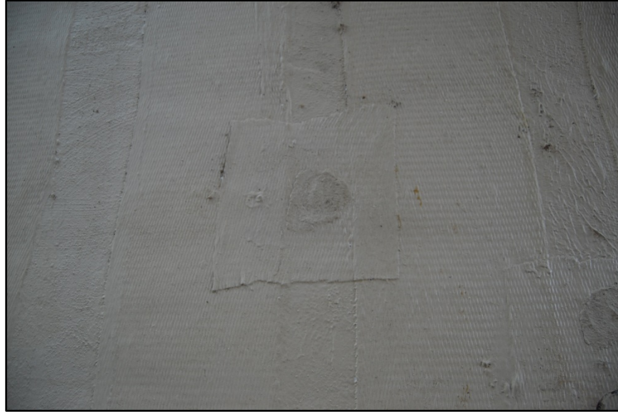
Figure B.14 CFRP patching.
