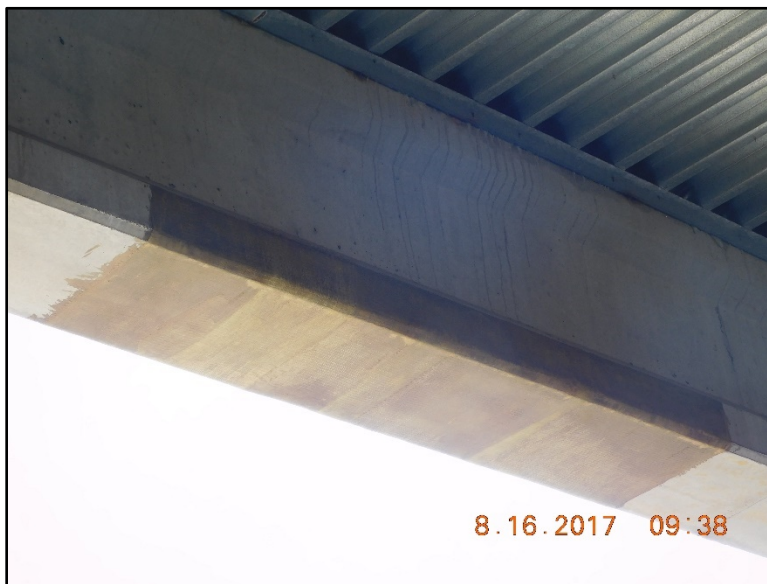
Figure B.107 Repair from underside of 116th Street Bridge.
