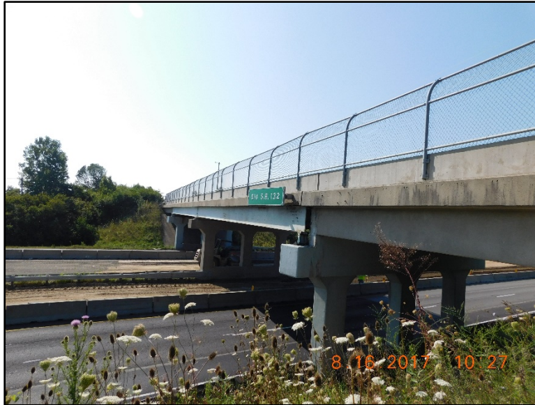
Figure B.108 Panoramic view of the bridge facing southeast.
