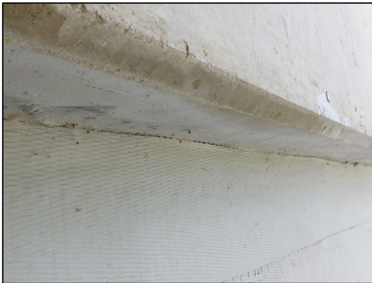
Figure B.87 Termination of wrap at pier cap.
