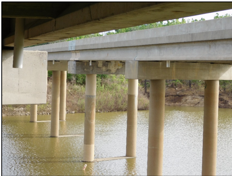
Figure B.71 Pier 4 Repairs on northbound bridge.
