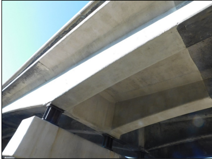
Figure B.140 Wrapped girders, diaphragm, and deck portion in northern span.
