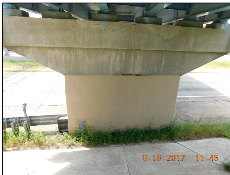
Figure B.115 Wrapped column at northern pier.
