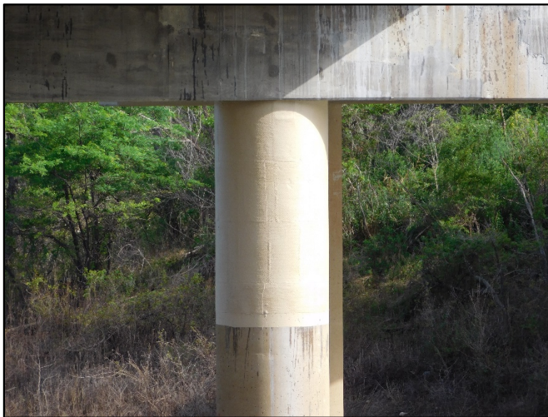
Figure B.73 Top of column repaired on southbound Pier 4.
