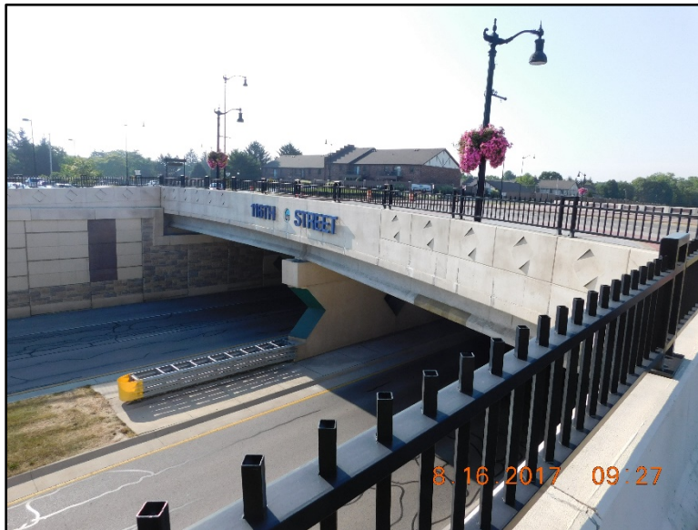
Figure B.102 Panoramic view of the bridge facing southeast.
