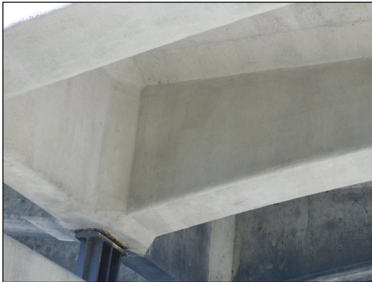
Figure B.141 Detailing of FRP repair at girder-diaphragm intersection.
