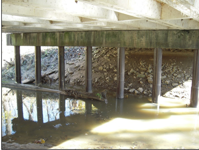
Figure B.150 FRP wraps on steel-encased columns of eastern pier.
