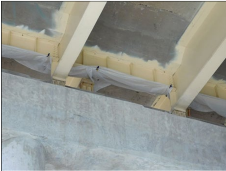
Figure B.191 Sealing of deck joint to prevent leaking onto pier.
