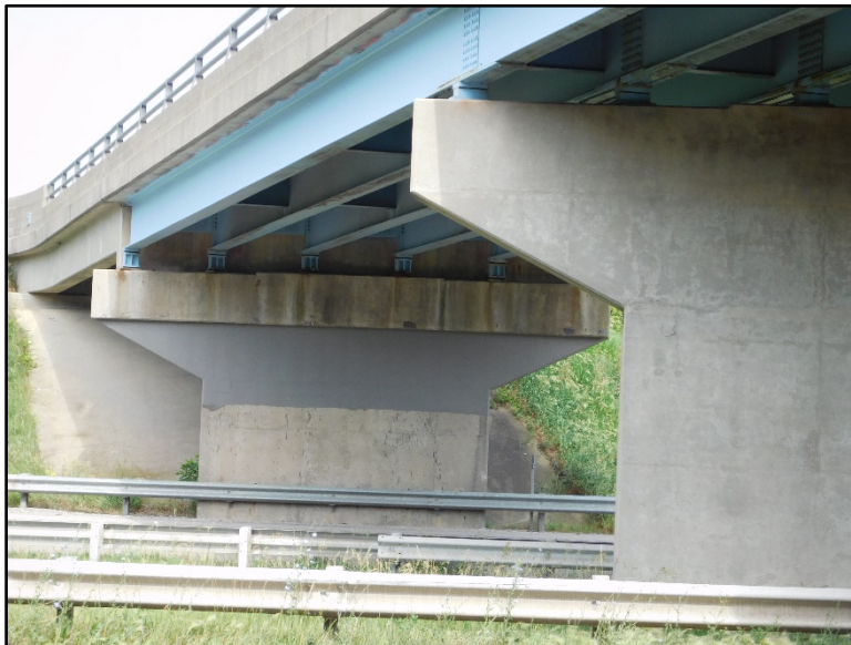
Figure B.38 View of bridge and FRP-repaired pier facing west.
