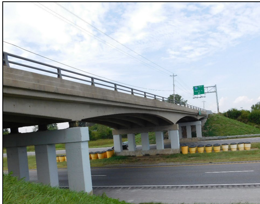
Figure B.128 Panoramic view of the bridge facing southeast.
