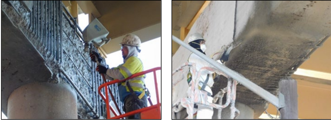
(a) (b) Figure B.184 Application of shotcrete to pier cap.
