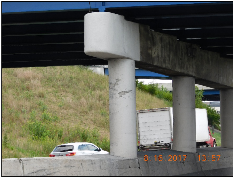
Figure B.125 Wrapped northernmost column and beam cap edge.
