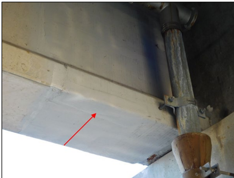
Figure B.166 Patching of FRP material.
