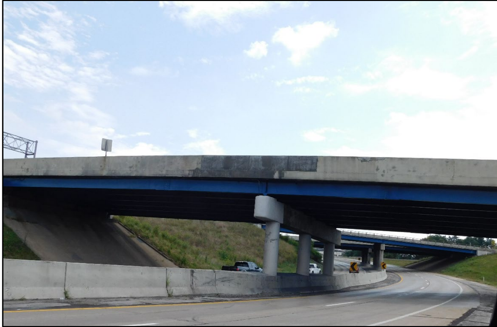
Figure B.122 Panoramic view of the bridge facing south.
