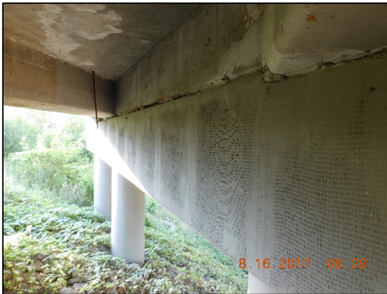
Figure B.98 Pier 4 wrapped beam cap and columns.
