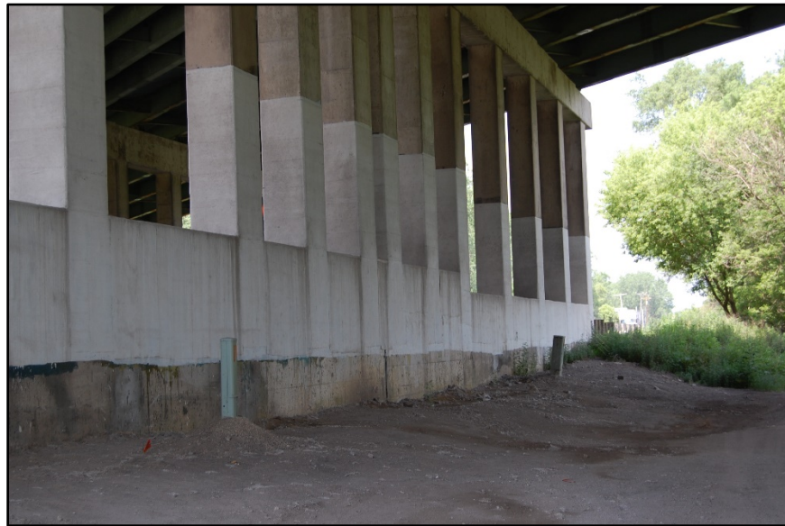
Figure B.21 Variable length of GFRP sheets on Bent 5 crashwall.
