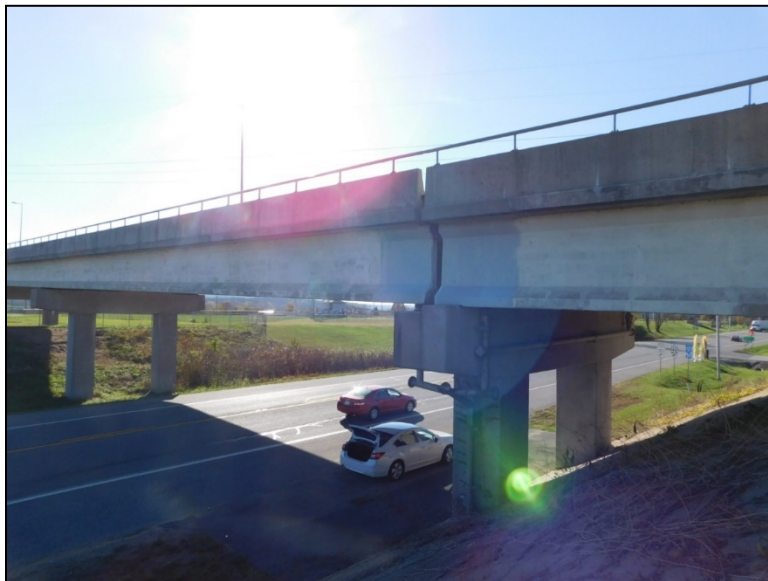
Figure B.155 Panoramic view of bridge spanning IN-156.
