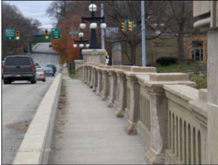
Figure B.7 East Side railing facing north (from Skinner (2011) inspection report).
