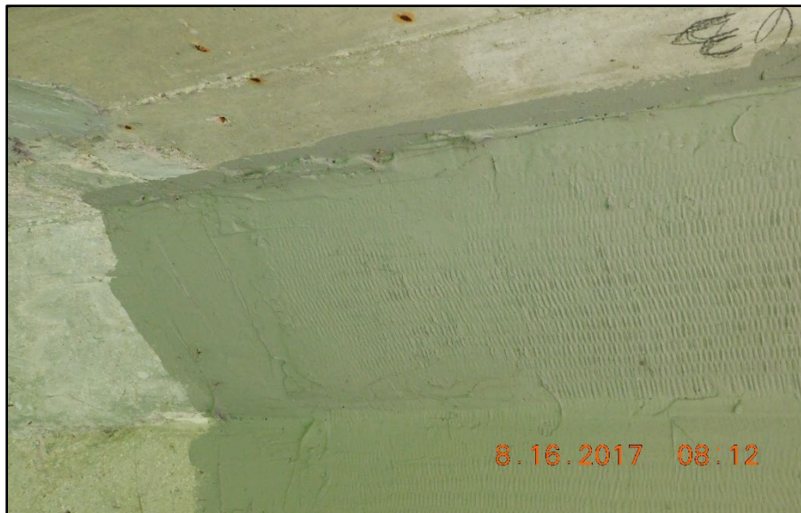
Figure B.94 Beam end wrapping up to deck.
