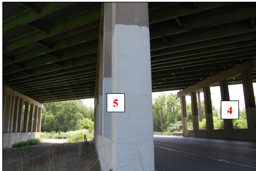
Figure B.18 View of both bents facing west.
