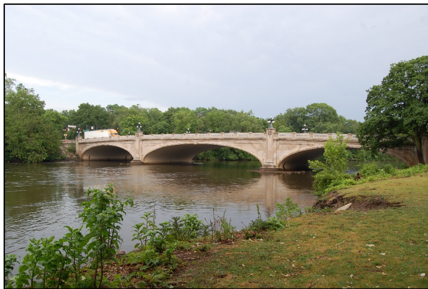
Figure B.5 Panoramic view of the bridge facing east.
