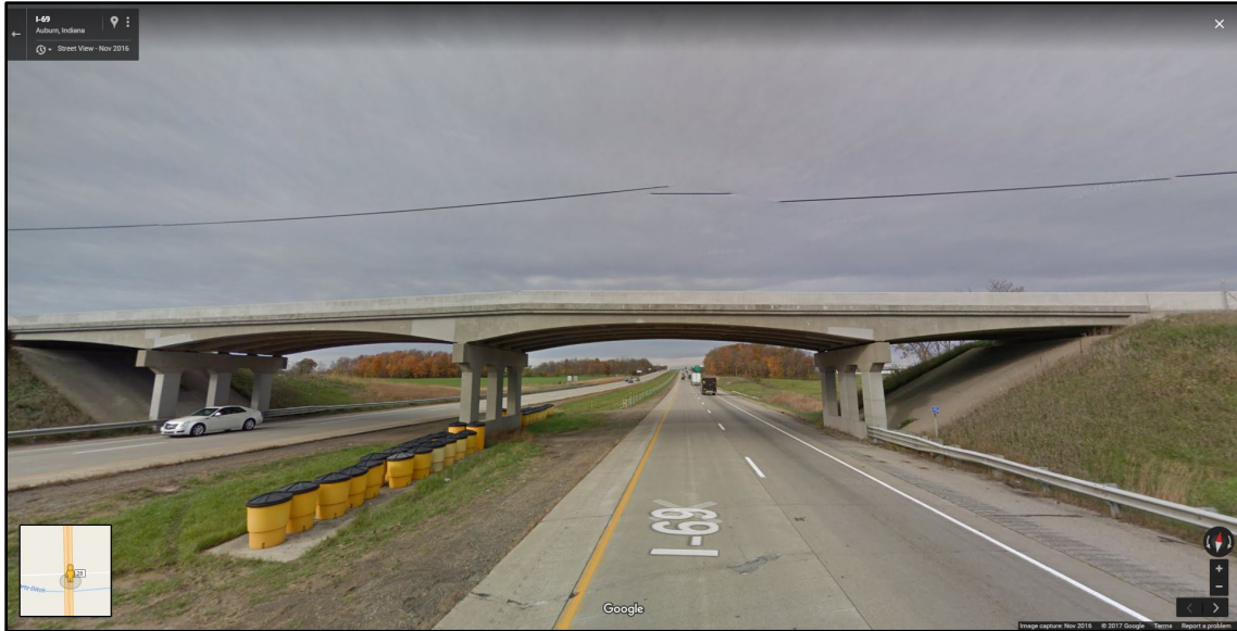
Figure B.27 Panoramic view of the bridge facing north (Google, 2016).
