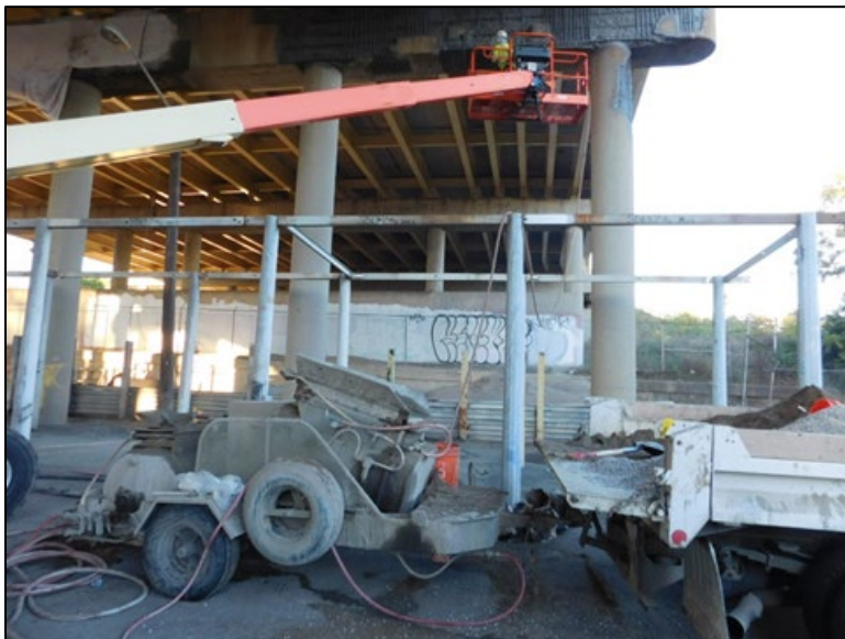
Figure B.183 Shotcrete material preparation station.
