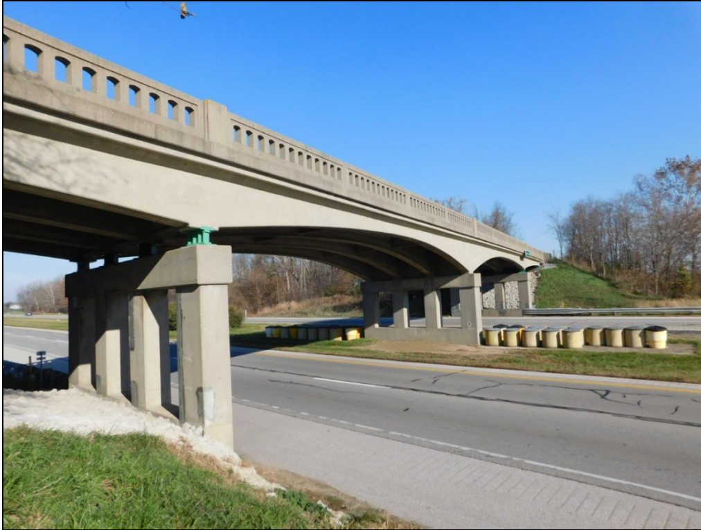
Figure B.169 Panoramic view of bridge.
