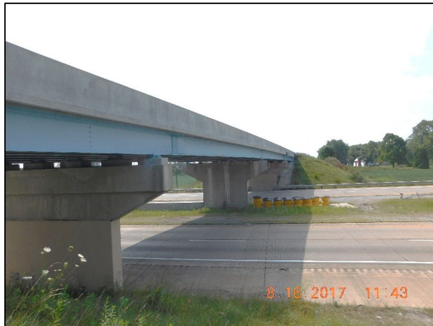
Figure B.114 Panoramic view of the bridge facing Southeast.
