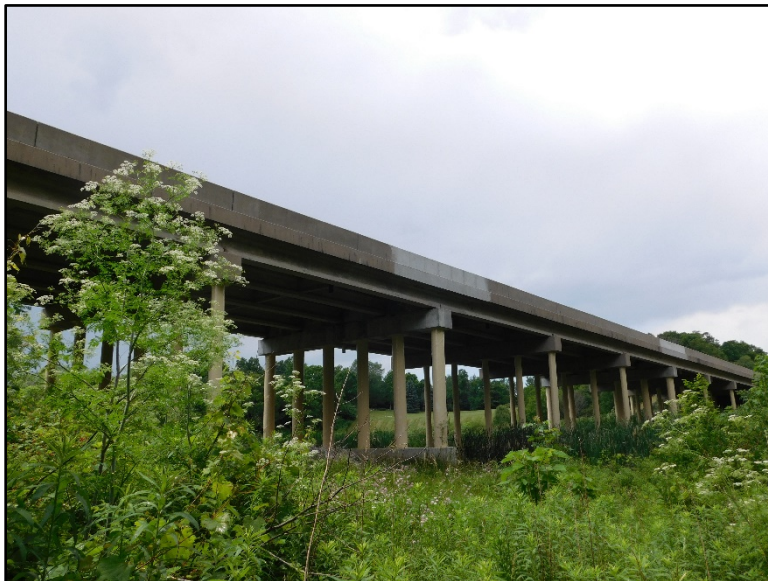
Figure B.45 Panoramic view of the bridge facing west.
