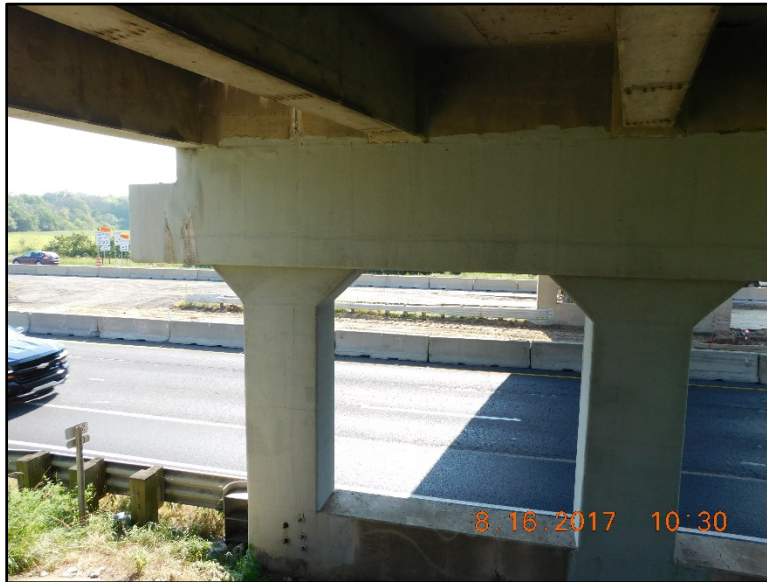
Figure B.109 Wrapped columns and pier cap at northwestern pier.
