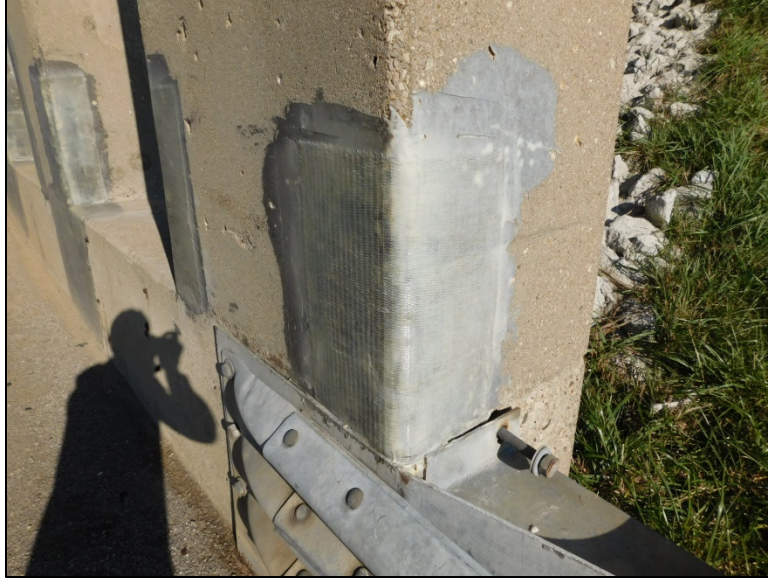
Figure B.172 Corner patching of columns at northern pier.
