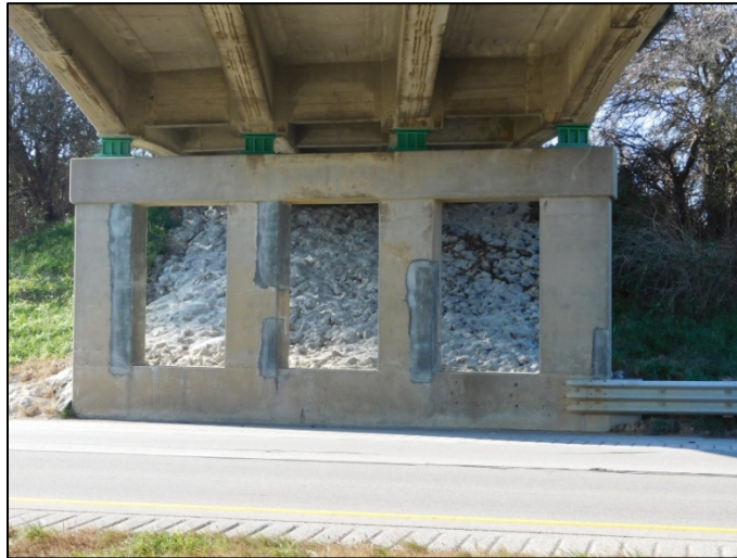
Figure B.170 Southern pier FRP patching.
