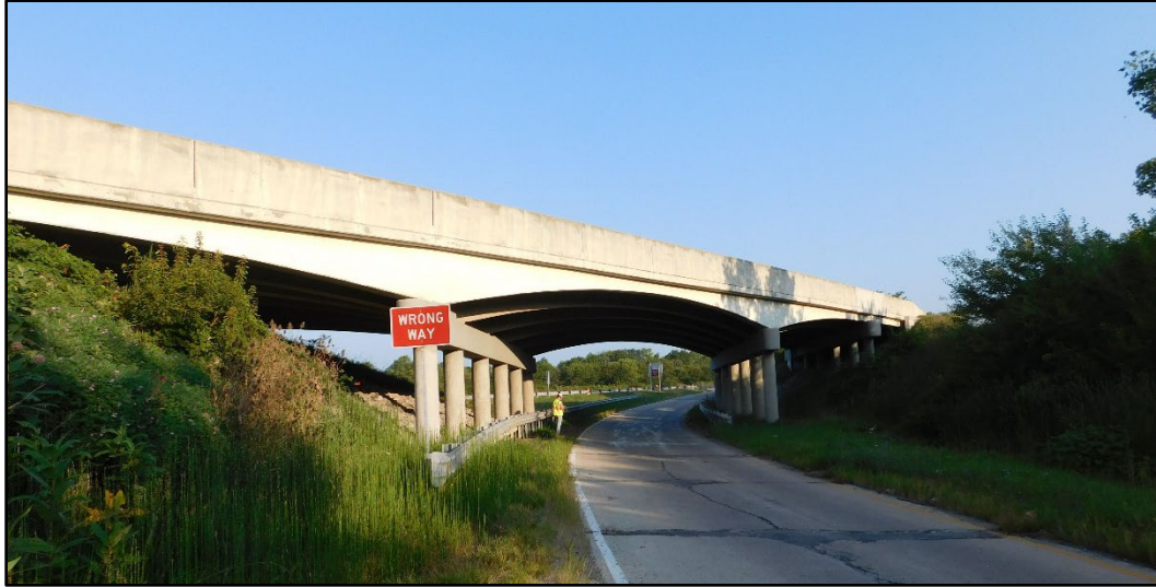
Figure B.88 Panoramic view of bridge facing west.
