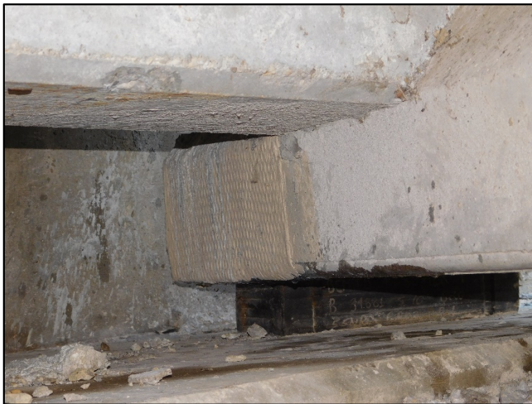
Figure B.75 Interior beam end repair (sheet termination at diaphragm).
