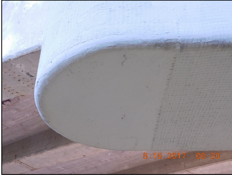
Figure B.97 Termination of pier cap wrapping at edge of cap.
