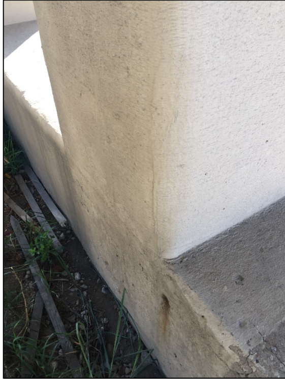
Figure B.142 Column wrap terminated at top of crashwall.
