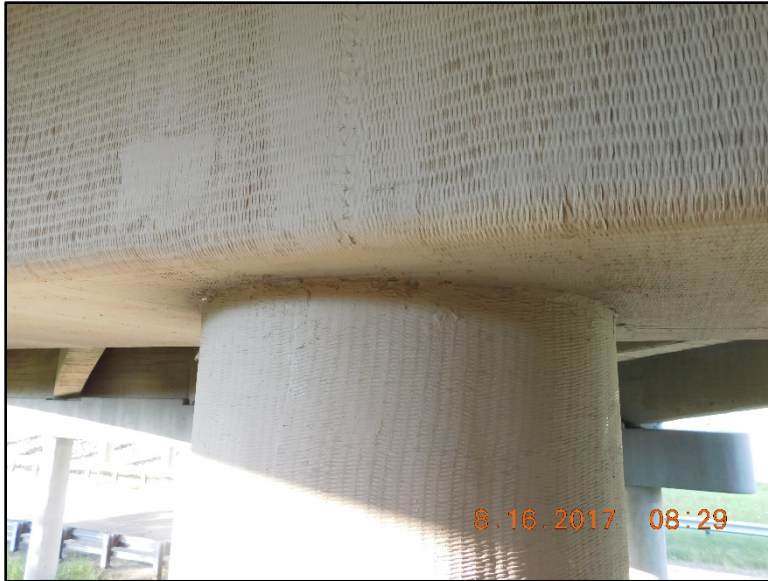
Figure B.99 Pier cap-column joint.
