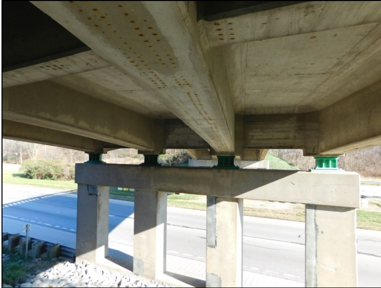
Figure B.174 View of entire pier and beam ends.
