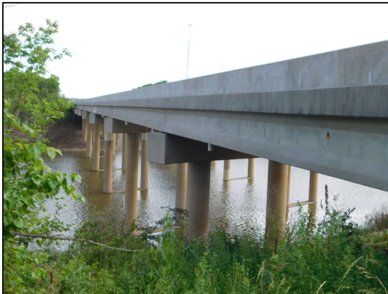
Figure B.61 Panoramic view of the southbound bridge facing northeast.
