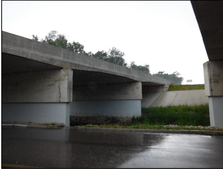
Figure B.76 View of the US 30 eastbound bridge facing southwest.
