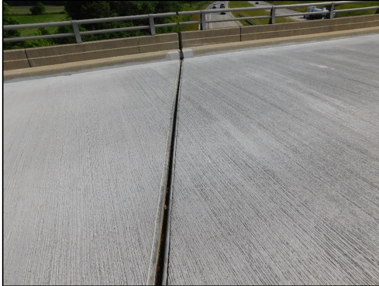
Figure B.44 Joint and deck surface directly above repaired pier.
