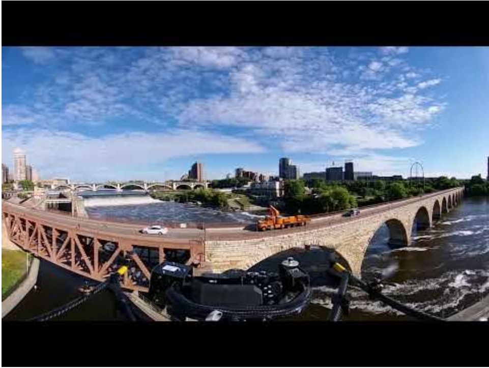
Figure 4-28 Video of Falcon 8+ Performing Inspection
