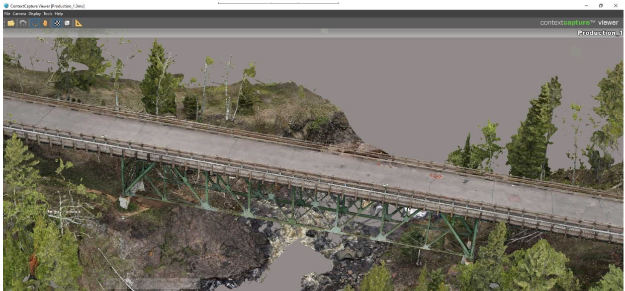
Figure 4-24 Tettegouche Bridge Modeled in Context Capture
