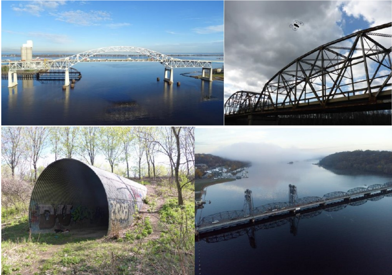
Figure 1-2 Overall Photograph of Four Bridges Selected for Phase II UAS Inspection
