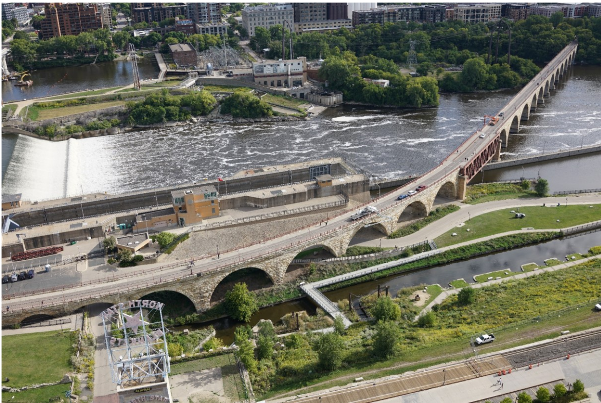
Figure 4-26 Overall Photo of the Stone Arch Bridge
