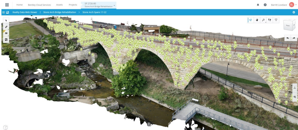
Figure 4-32 Reality Model of Spans 17-22 With Inspection Notes
