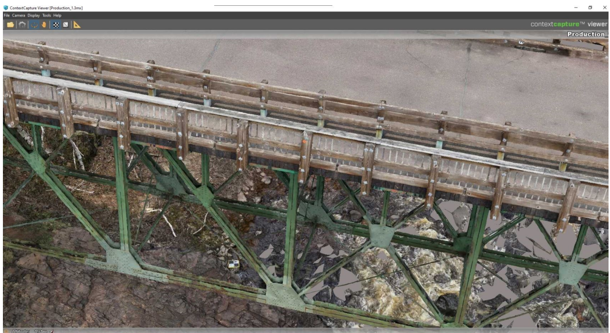
Figure 4-25 Tettegouche Bridge Context Capture Model Close Up View
