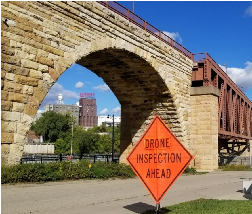
Figure 1- 3 Drone inspection ahead sign at the Stone Arch Bridge in Minneapolis.
