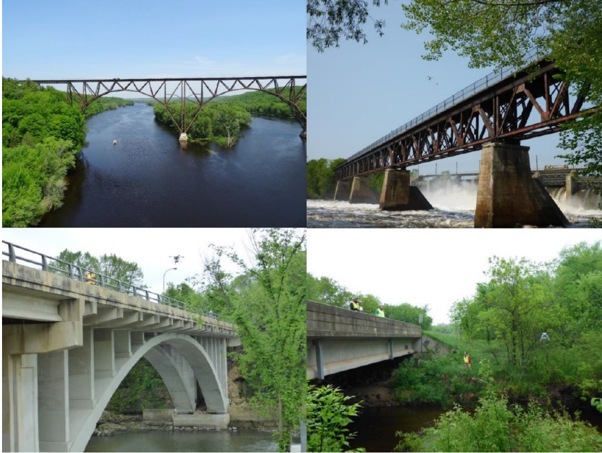
Figure 1-1 Overall Photographs of Four Bridges Selected for Phase I UAS Inspection (Shown clockwise from upper right, Arcola Bridge, Morrison County Pedestrian Truss, Chisago County Bridge, Oronoco Concrete Arch)
