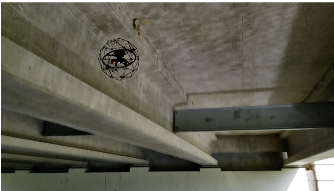
Figure 1- 1 View of Flyability Elios under a bridge
