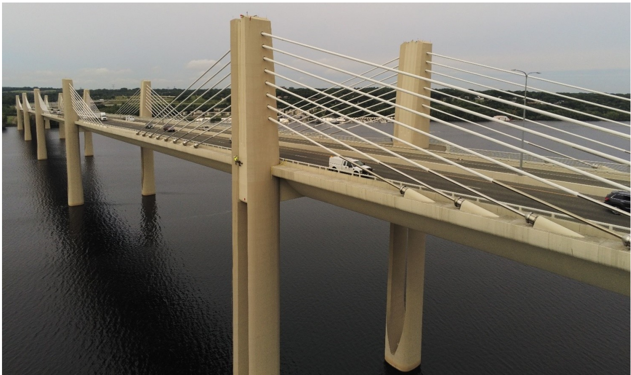
Figure 4-1 St. Croix Crossing Bridge
