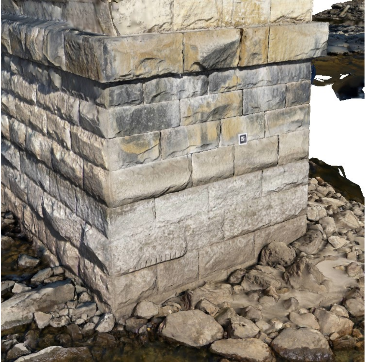
Figure 4-34 Reality Model Zoomed in to Pier During River Drawdown
