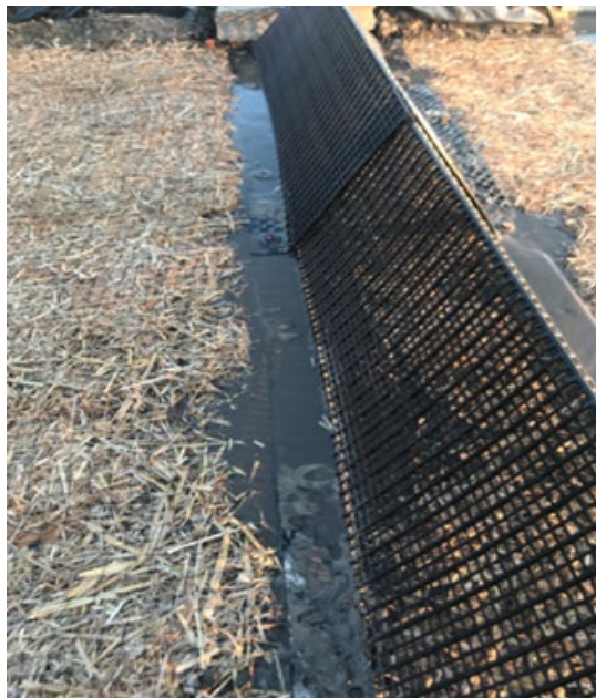
B. GeoRidge slowed down water velocity
