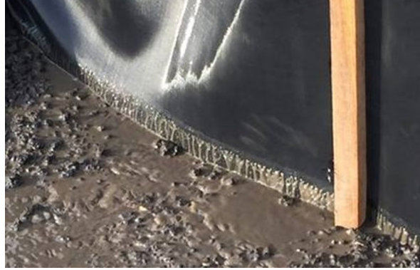
Figure 26. Photo. Woven monofilament geotextile flow.
