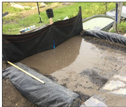
Figure 1. Photo. Silt fence (IDOT-approved fabric).
