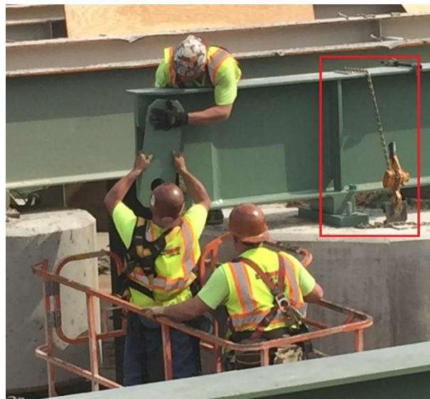
Figure 2-38. A chain-down system anchored to substructure (Photo courtesy: MDOT)
