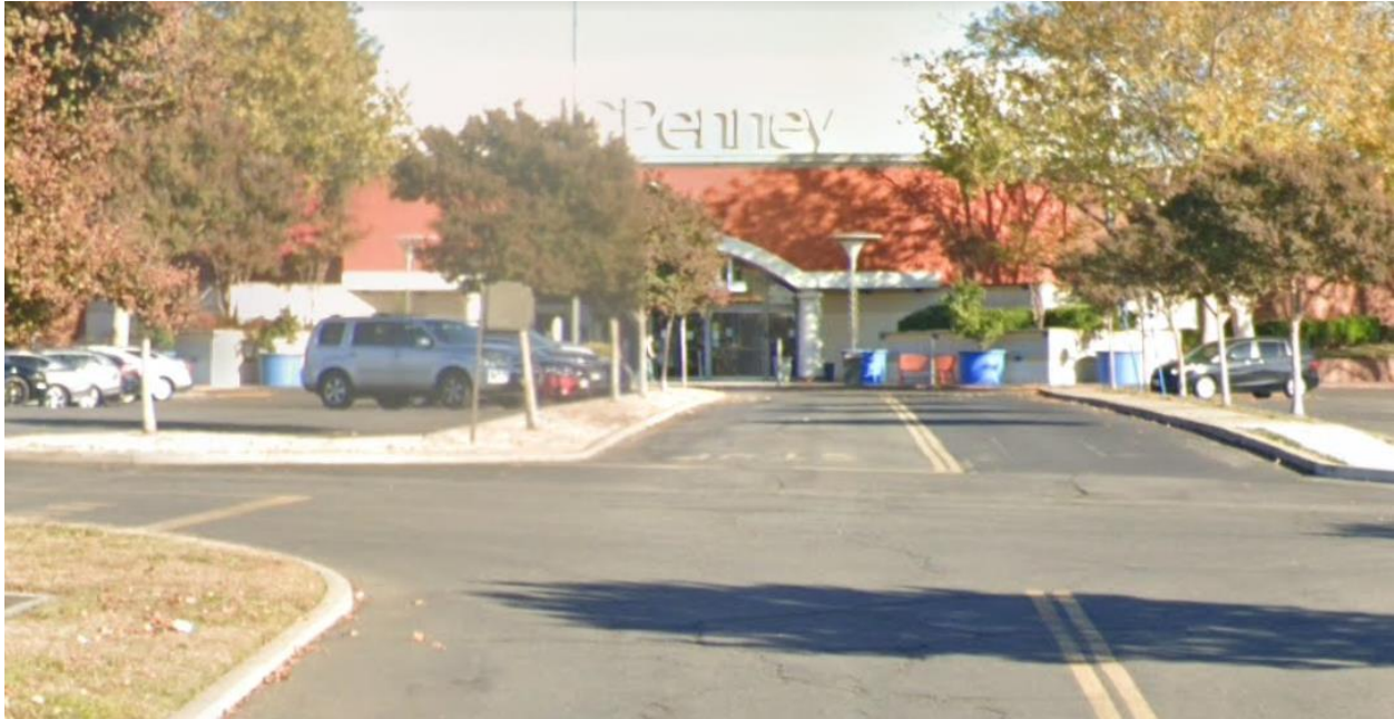
Figure 11.3. View of Internal Road leading to JCPenney in Sunrise Mall. (Google Earth, 3/22/2021)
