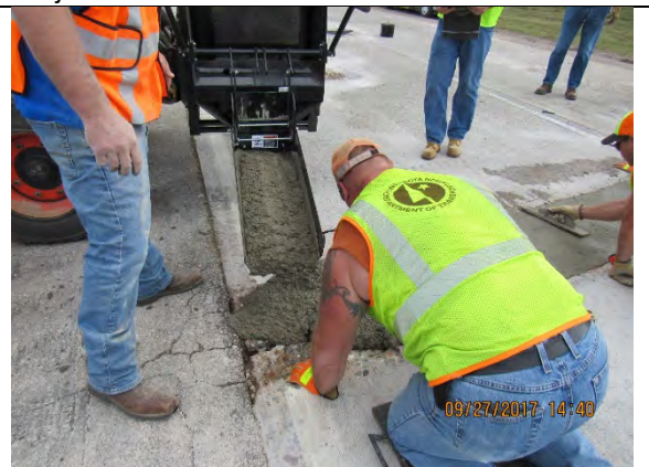
Photograph: 94003 (A) Western Material and Design, FasTrac246 Subject: Concrete placement
