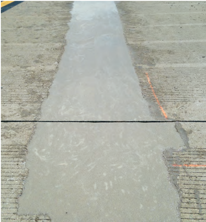
PaveSaver™ Airfield Repair Application
