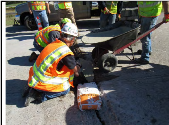
Photograph: 94001 – CTS, Rapid Set DOT Repair Mix Subject: Placing mixture
