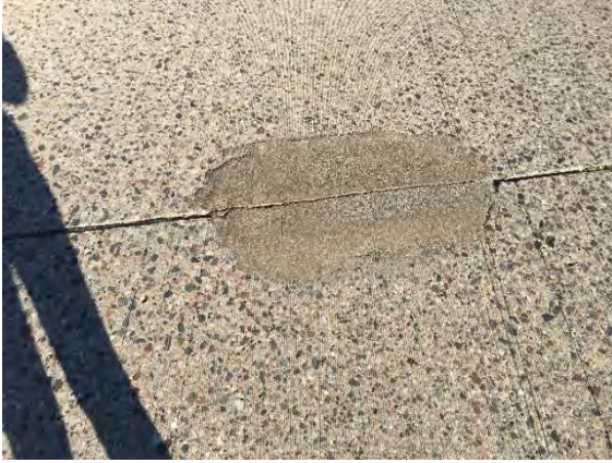
Figure 4.2 Patch Condition Rating = 4 [No Distress]
