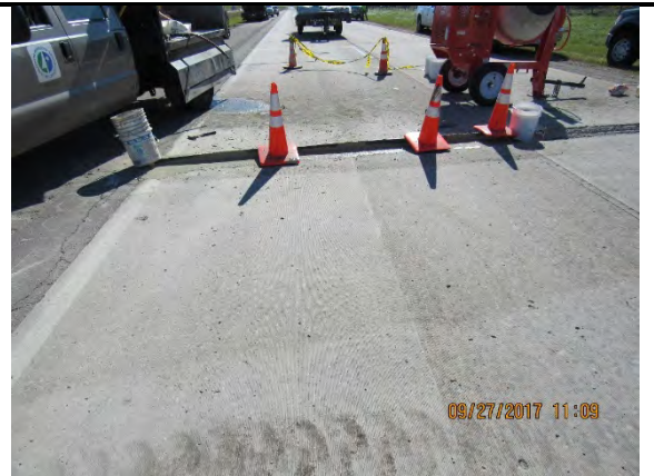
Photograph: 94001 – CTS, Rapid Set DOT Repair Mix Subject: Weighing down foam board
