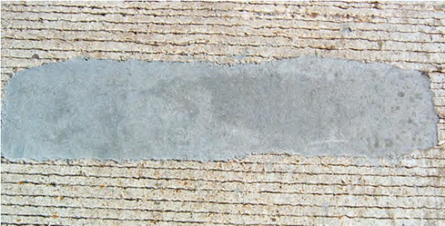
Top and Center images: Highway Spall Repair, Highway 99, Fort Bend County, TX.
