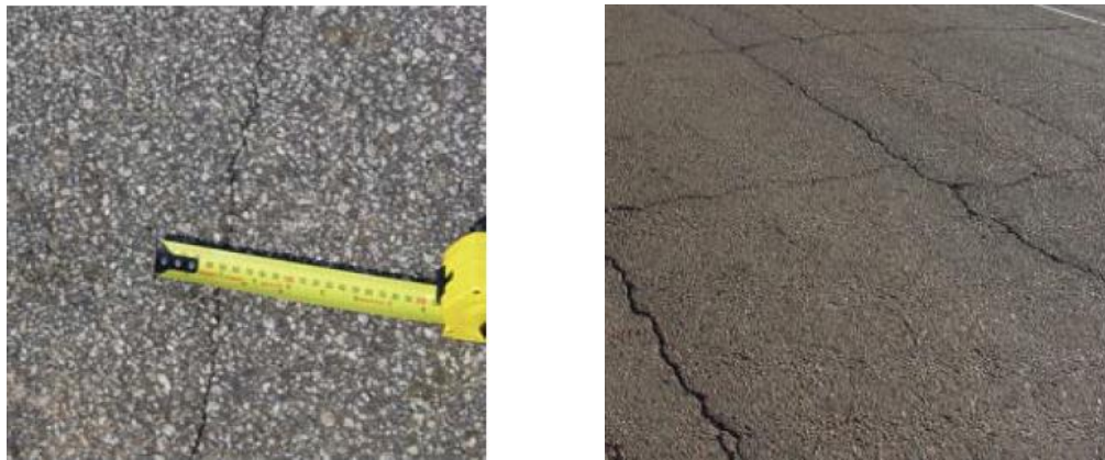
Figure 10: Reflective cracking in flexible pavement due to underlying soil cement base [13]
