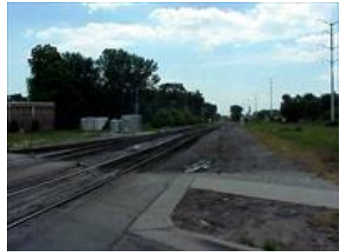
Figure 18. E 137 th RR Crossing
