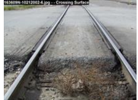
Figure 24. Perry Ave. RR Crossing
