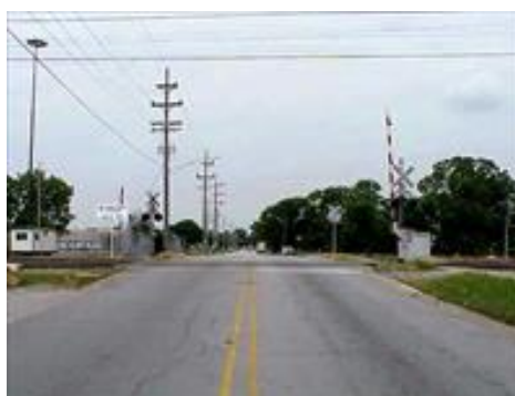
Figure 15. E 144 th St. RR Crossing
