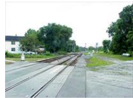
Figure 9. Lincoln Ave. RR Crossing
