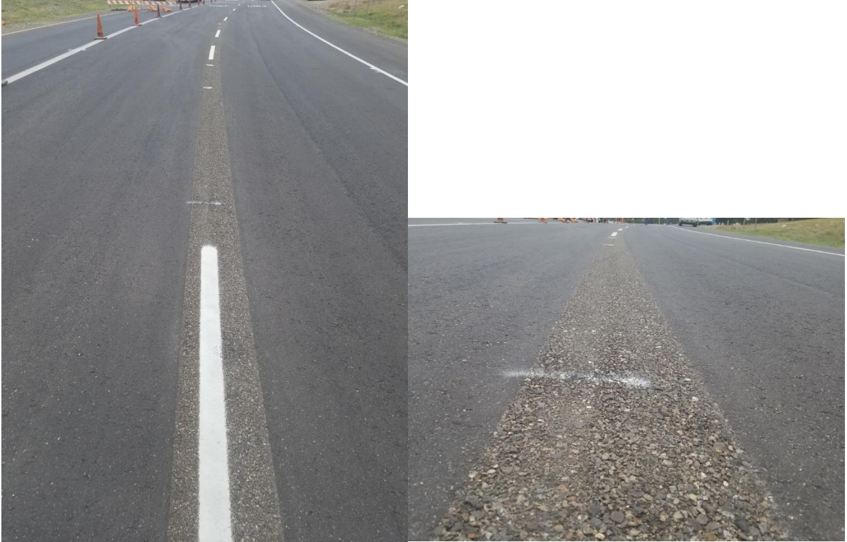
Figure 38. High-Pressure Water Blasting on Asphalt.
