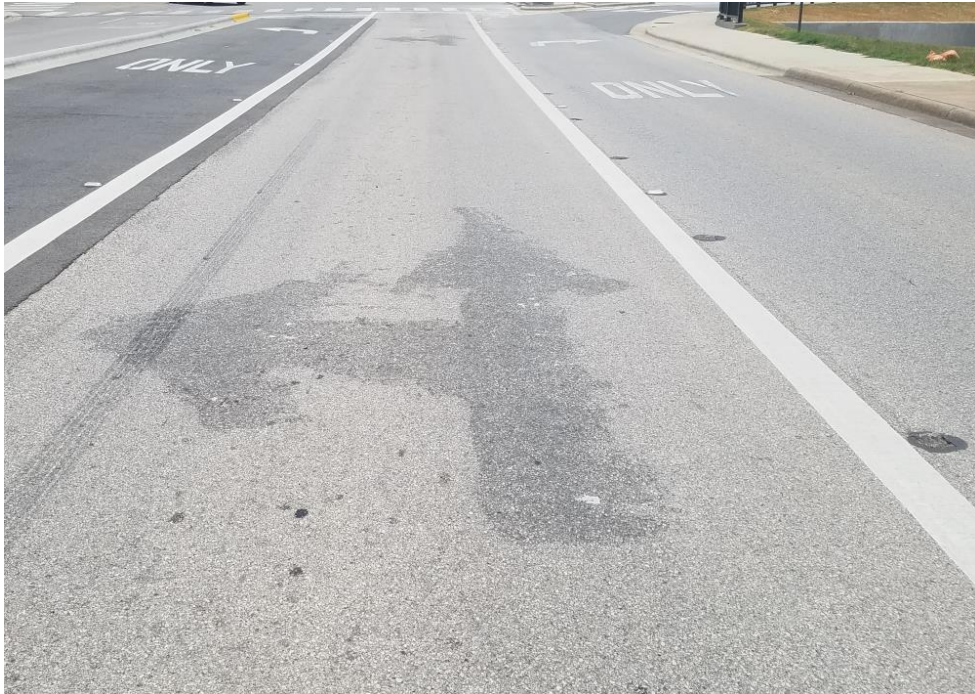
Figure 39. Hand-Operated Flailing Removal on Asphalt.
