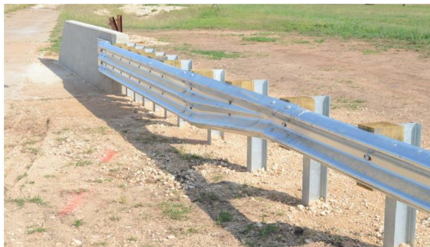
Figure 2.8. Thrie Beam Transition without Curb.
