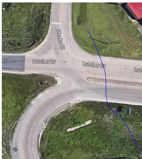
Figure 50. IH 10 Service Frontage Road Intersection with Meeks Dr. and WB IH 10 Exit Ramp.
