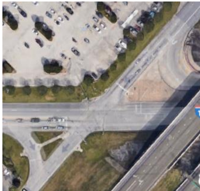
Figure 52. WB/SB IH 10 Service/Frontage Road Intersection with Washington Boulevard.
