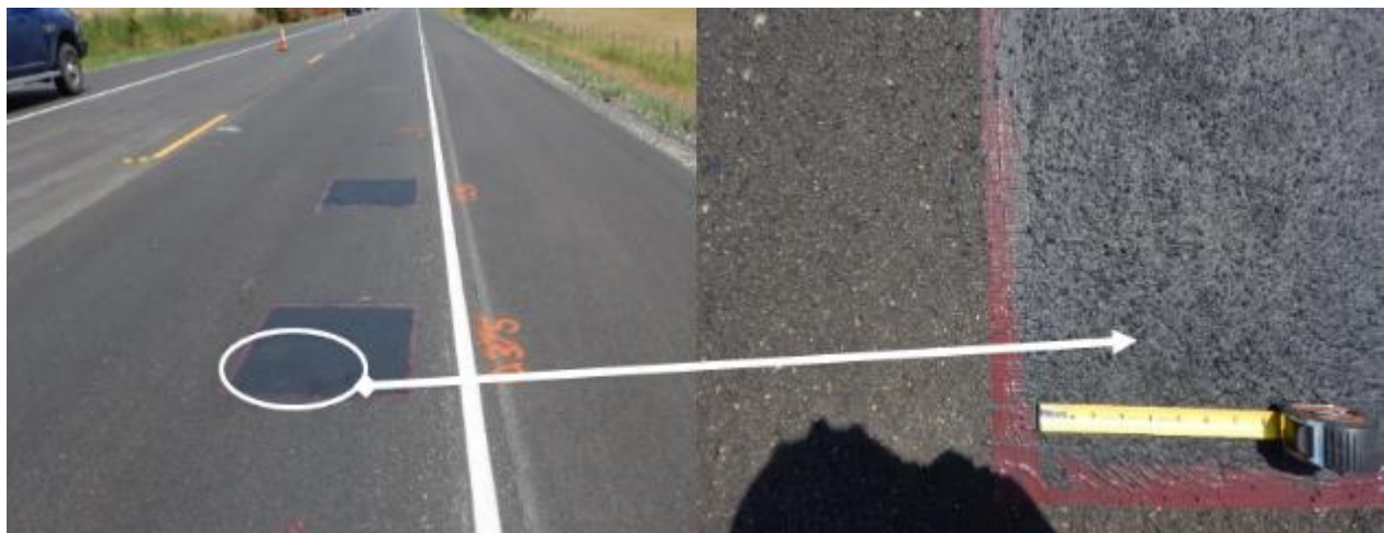
Figure 32. UTSS Treated Sections on SH 36.
