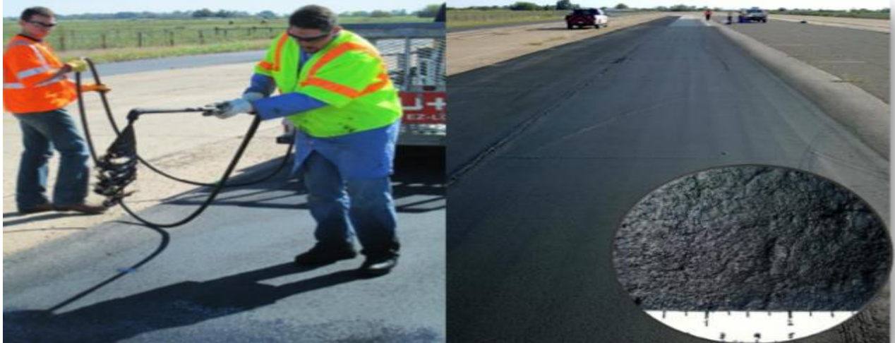
Figure 3. Application of UTSS (TTI Riverside Facility).
