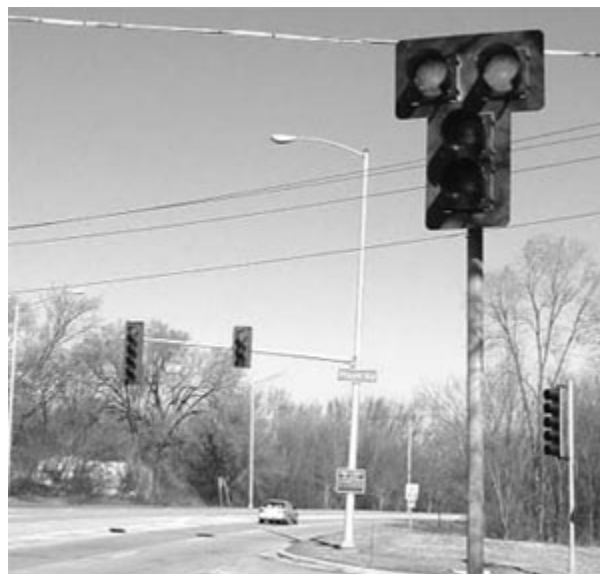
Figure 9. Photo of signal head using a double red signal indication.
