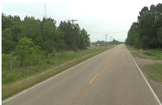
Figure 4. Overall condition of inverted section on LA 97 in 2017.
