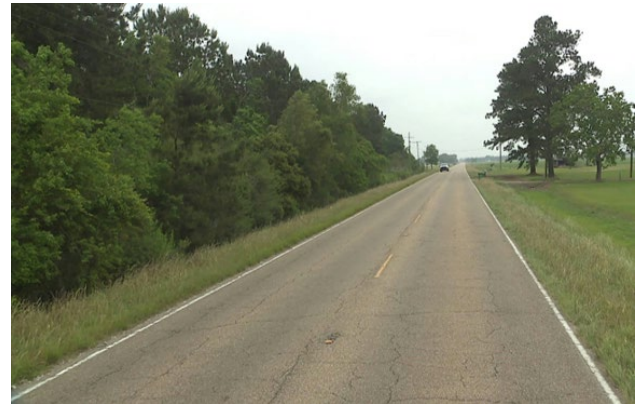
Figure 1. Reflective shrinkage cracks in the form of block cracking on LA 97.
