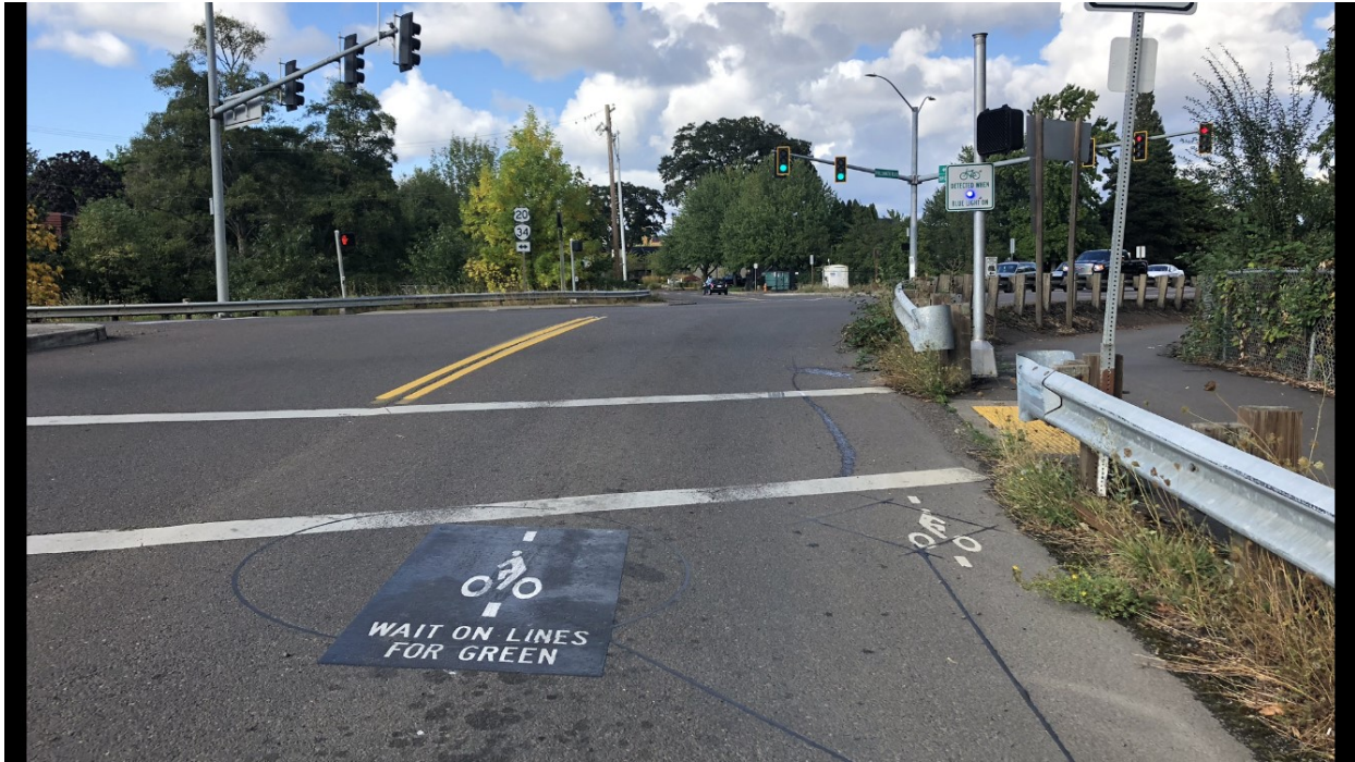
Figure 6.5 Blue detection confirmation light embedded in sign, placed nearside
