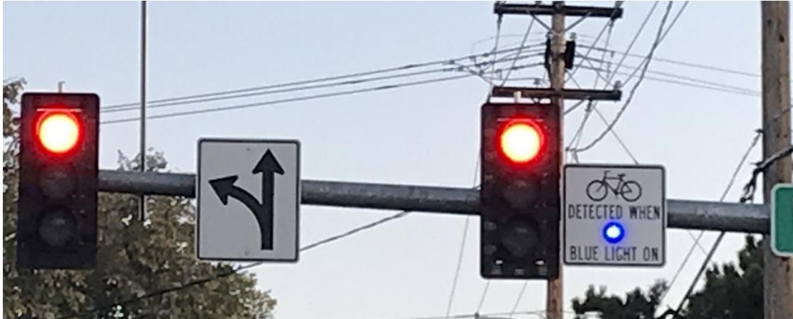
Figure 6.2 Blue detection confirmation light embedded in sign
