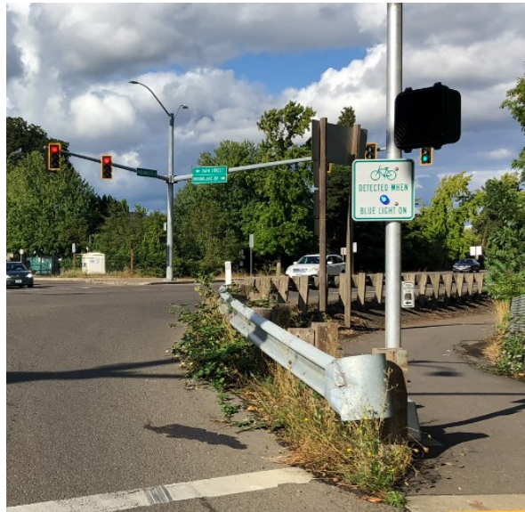
Figure 3.4: Blue detection confirmation light in embedded in supplemental sign, nearside
