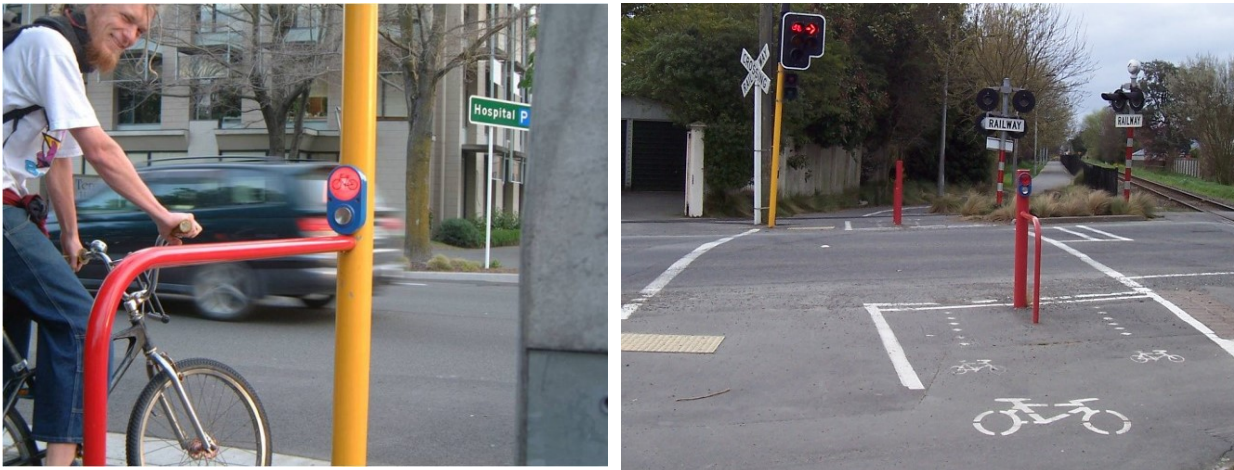
Figure 2.15: Nearside confirmation system in Christchurch, NZ (Source: G. Korrey)
