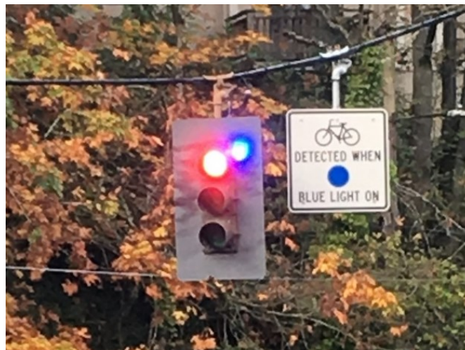
Figure 3.2: Blue detection confirmation light in backplate with supplemental sign, farside
