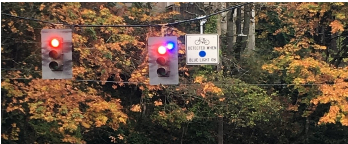
Figure 6.1 Blue detection confirmation light in back plate with sign
