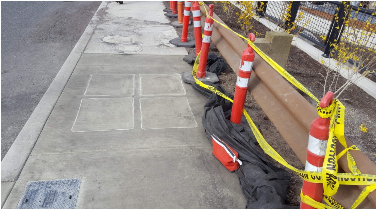
Figure 3.3: SLAB detector at Colorado Avenue in Bend MPO
