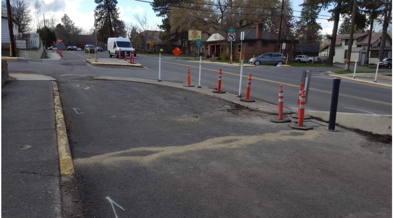
Figure 3.1: Separated inductive loop detector at Franklin Avenue in Bend MPO
