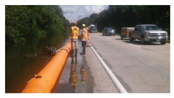
**Figure 1b.** The Louisiana Department of Transportation and Development (DOTD) checking water-filled barriers next to an evacuation route during March and August of 2019 flooding events. (Source: Louisiana DOTD)
