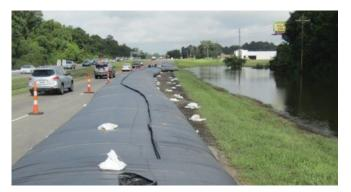
**Figure 1a.** The Louisiana Department of Transportation and Development (DOTD) successfully used water-filled barriers to manage flood impacts and maintain mobility during flood events in March and August of 2019. (Source: Louisiana DOTD)
