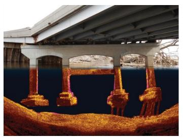
Figure 4. Underwater inspection of a Nebraska Route 13 bridge near Hadar included acoustic imaging that showed timber piles under the upstream footings were crushed or washed away. (Source: Nebraska Department of Transportation)
