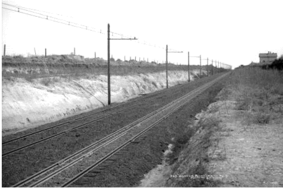
Figure 197. Cut-and-fill embankment on the Denver & Interurban Railroad between Denver and Boulder, c.1920 (current condition unknown). 773
