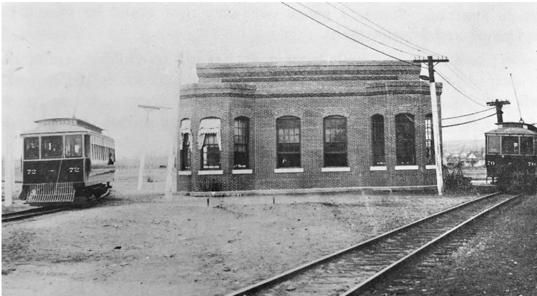
Figure 106. Clear Creek Substation east of West 52 nd Avenue and Wadsworth Boulevard. 512
