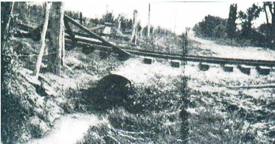
Figure 148. A corrugated culvert on the GJ&GRV interurban line to Fruita. 666
