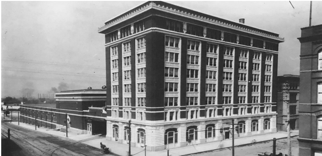
Figure 64. New Tramway central office building at 14 th and Arapahoe Streets with attached Central Division Car House, 1911. 333
