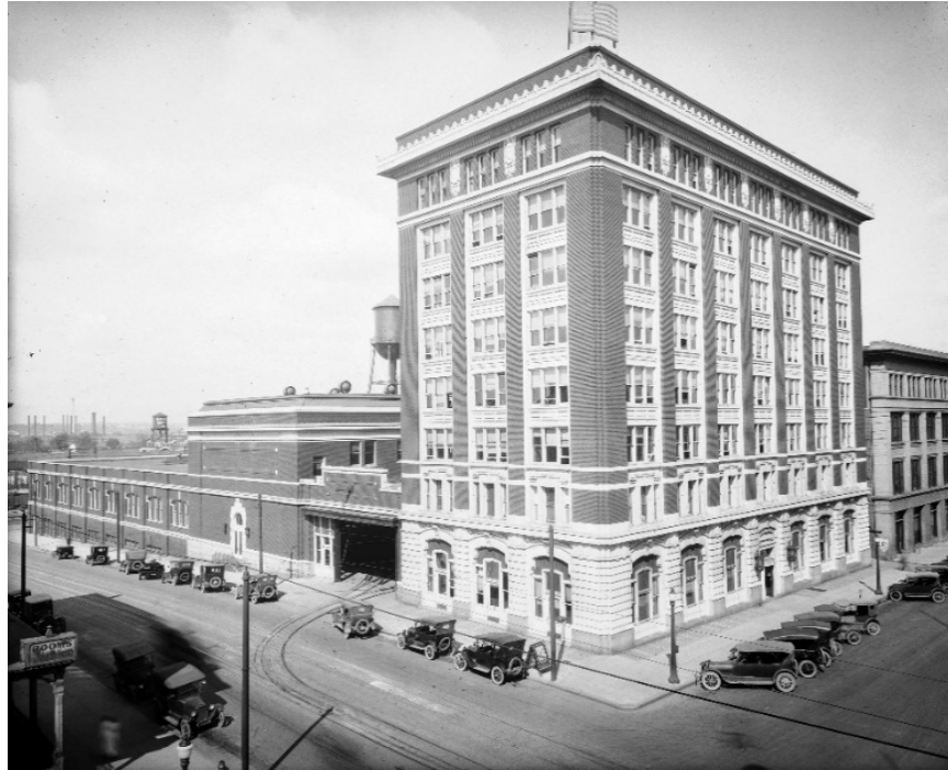
Figure 191. The extant Denver Tramway Building, c.1920. Carbarns are located behind the multi-story office building. 767
