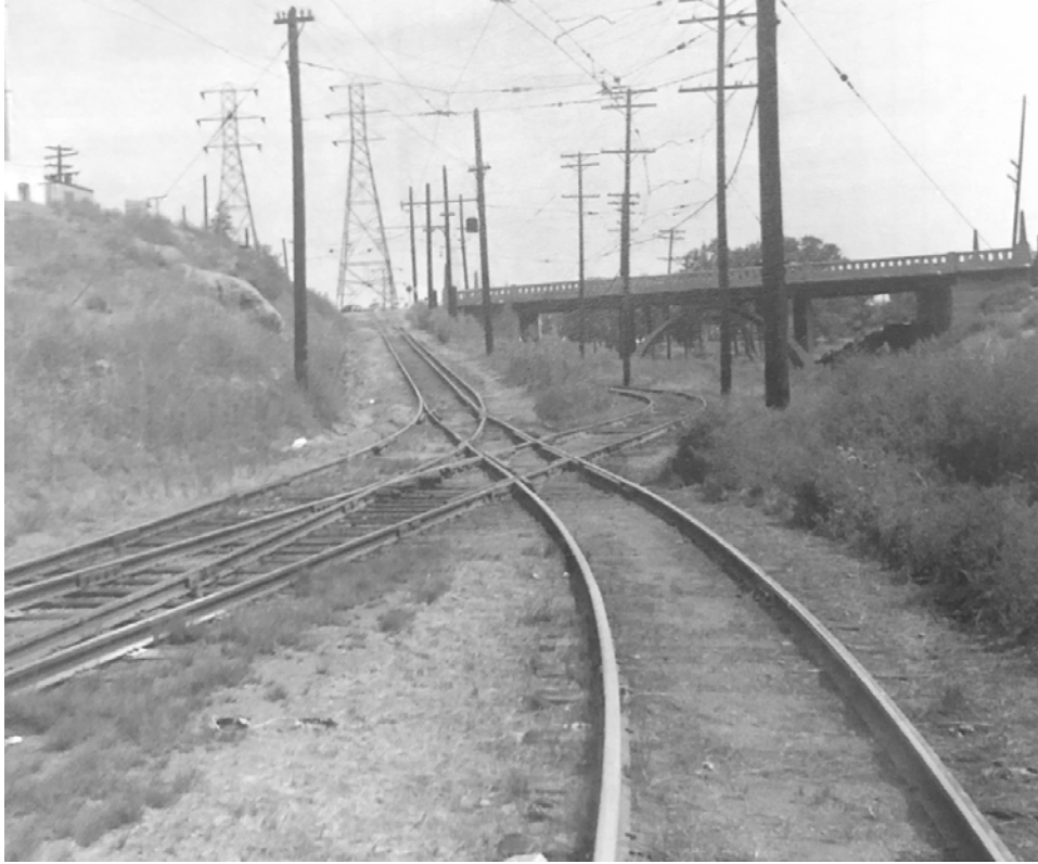
Figure 99. View of trackage at Barnum Junction looking east. 493
