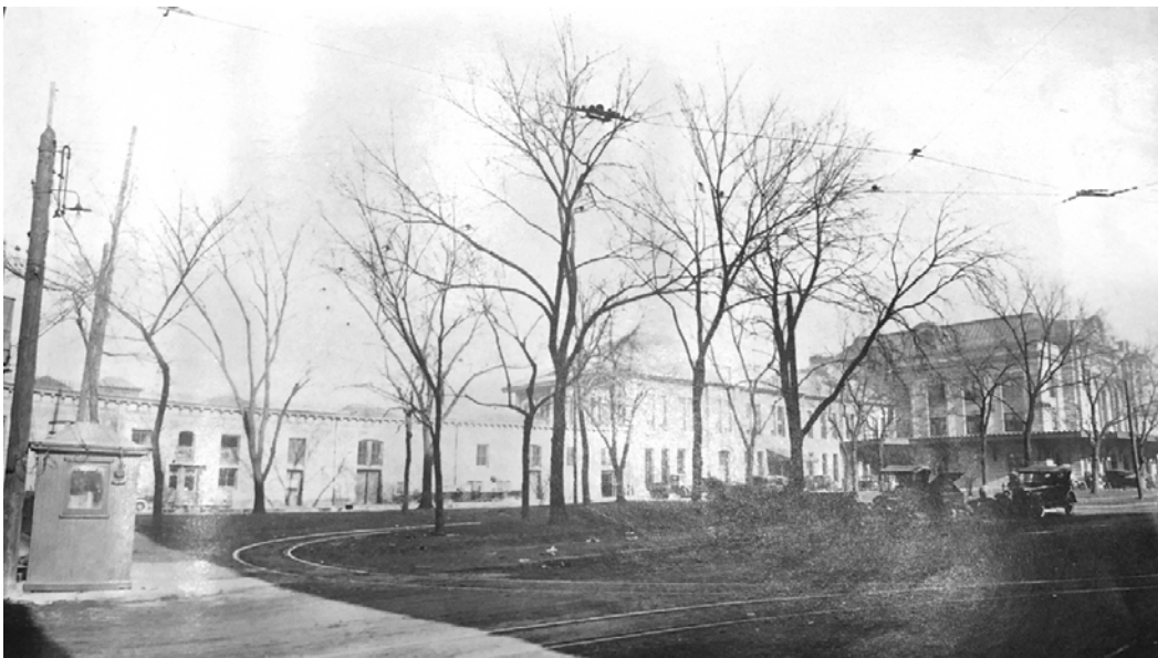
Figure 68. The loop at Union Station.
