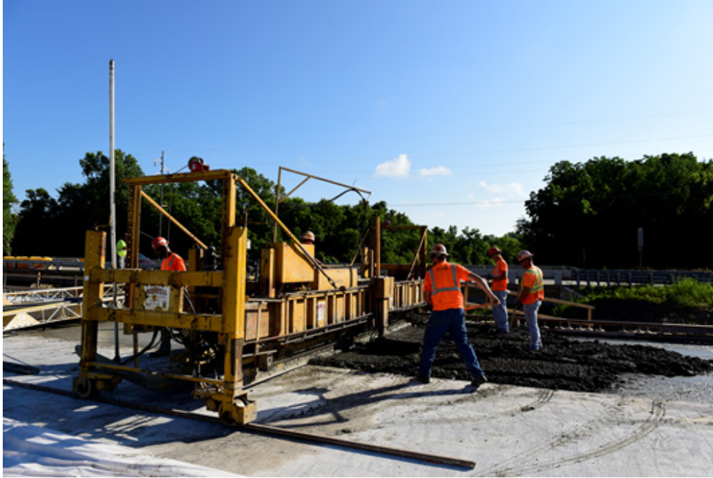
(a) Overlay concrete placement
