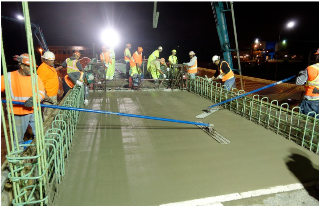
(b) Bull floating the north end of the deck
