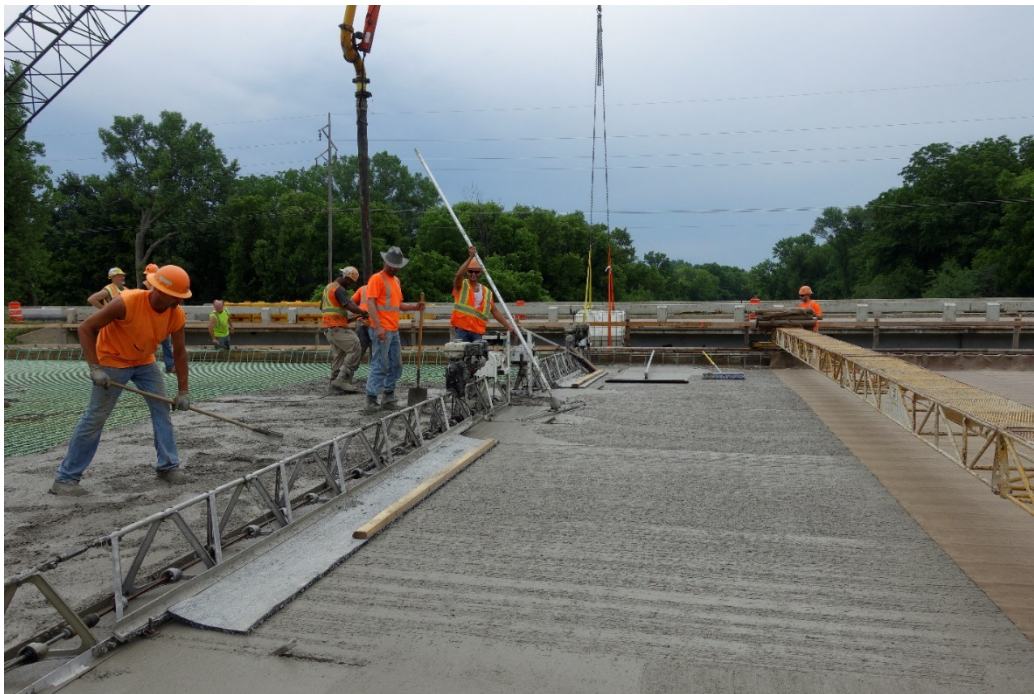
Figure 2.4: Placement, Finishing, and Curing Setup for IC-LC-HPC-2
