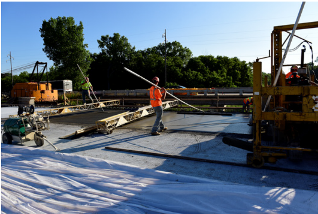
(b) Overlay concrete finishing
