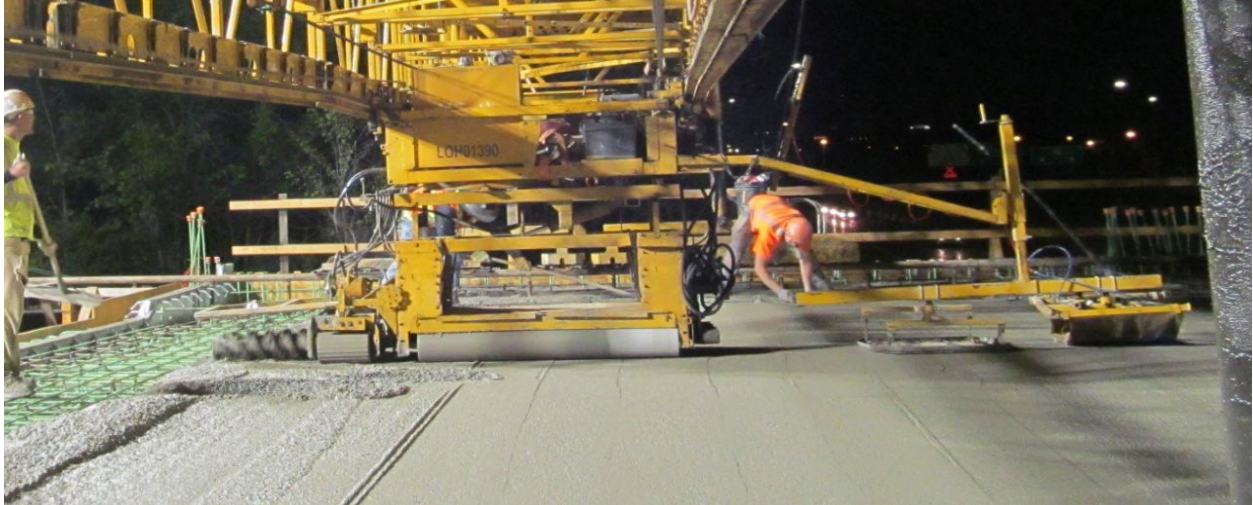
Figure 2.8: IC-LC-HPC-4 Finishing Equipment
