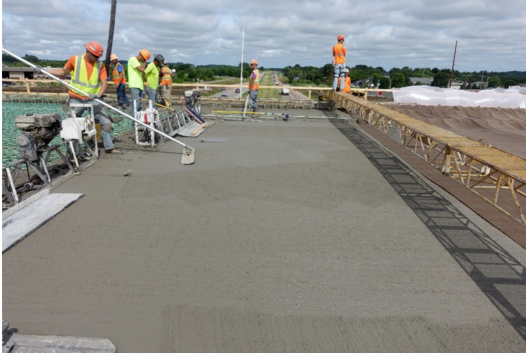
Figure 2.7: Placement, Finishing, and Curing Setup for IC-LC-HPC-3
