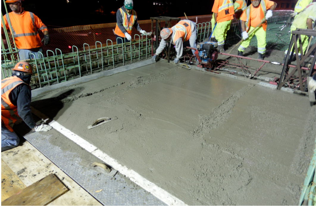
(a) Surface imperfections at the north end of the deck after first screed pass
