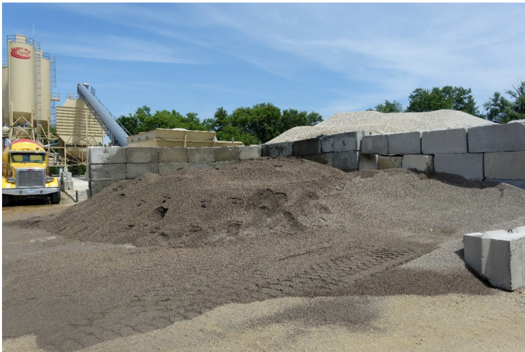
Figure 2.3: FLWA Storage for IC-LC-HPC-2 and IC-LC-HPC-3
