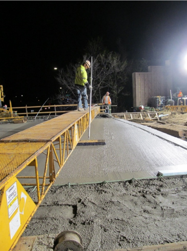
Figure 2.9: Consolidation and Finishing of IC-LC-HPC-4 Sidewalk Sections
