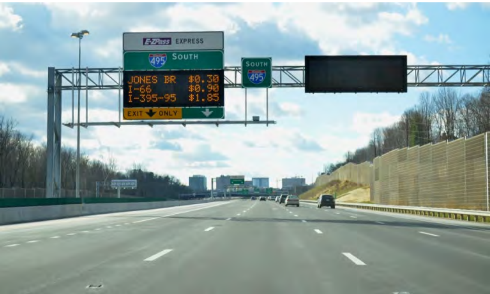
Figure 1-4. Demand-based roadway pricing has been implemented in Virginia in the form of high occupancy toll (HOT) lanes
