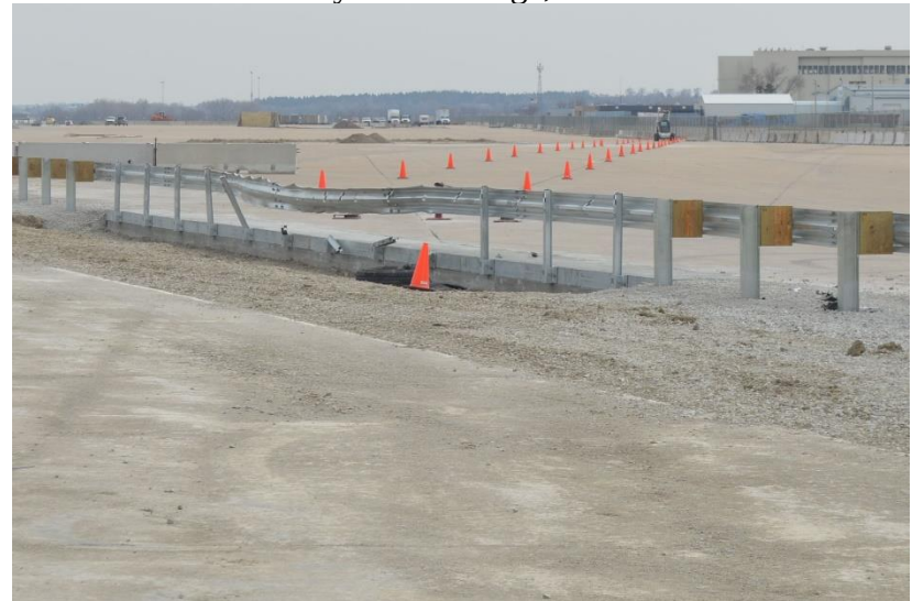
Overall System Damage, Downstream Behind View
