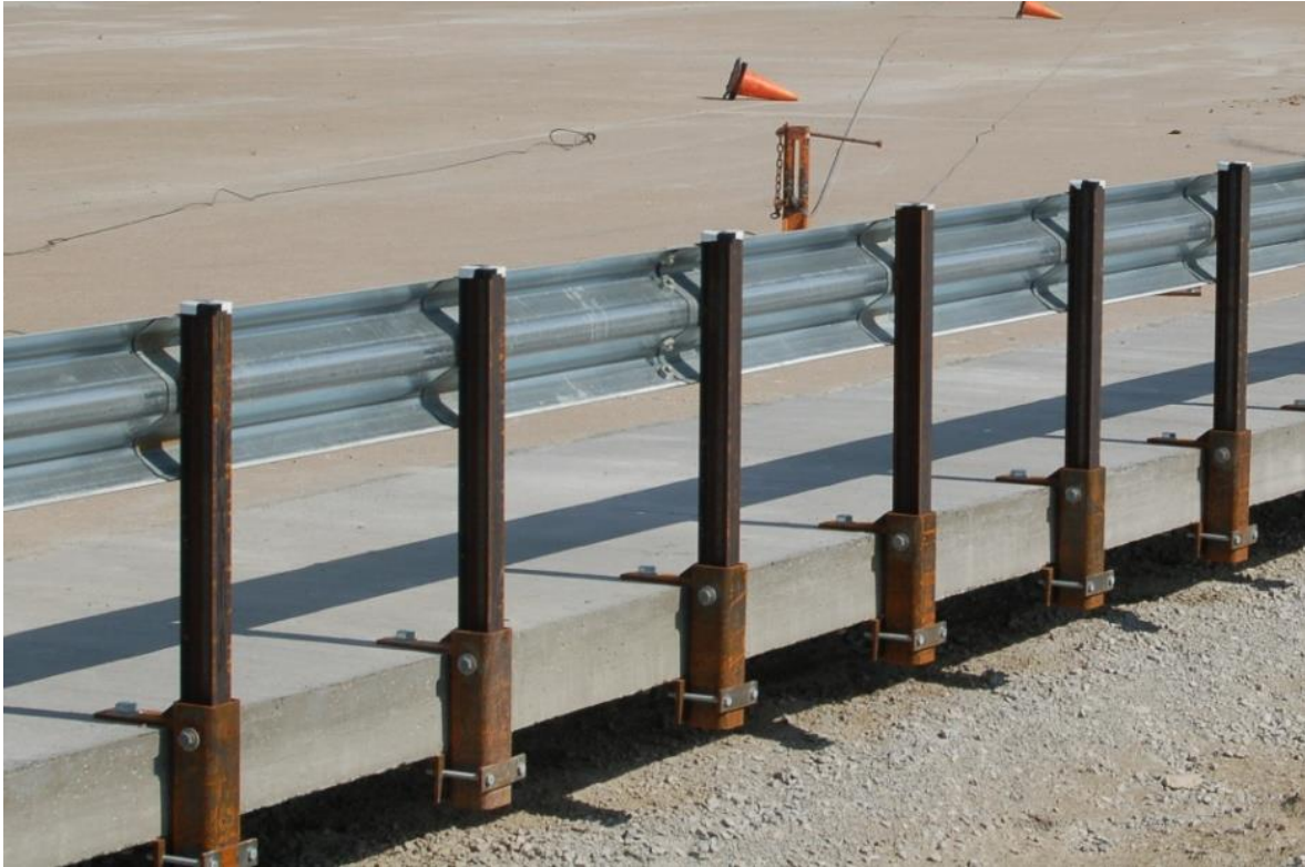
Figure 1. MGS Bridge Rail Test Installation [3]
