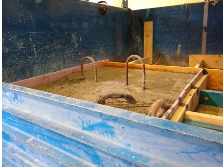
Figure 2.21: Concrete Slab during Pour and Compaction
