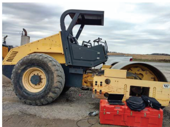
Figure 7.2 Bomag 211D-3 used for subgrade soil compaction.
