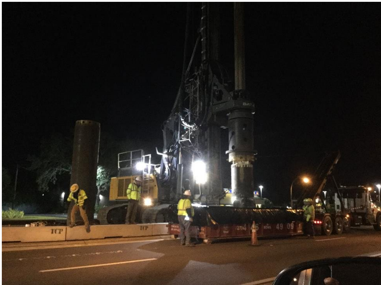
Figure 2-9. Drilling Test Shaft 3.
