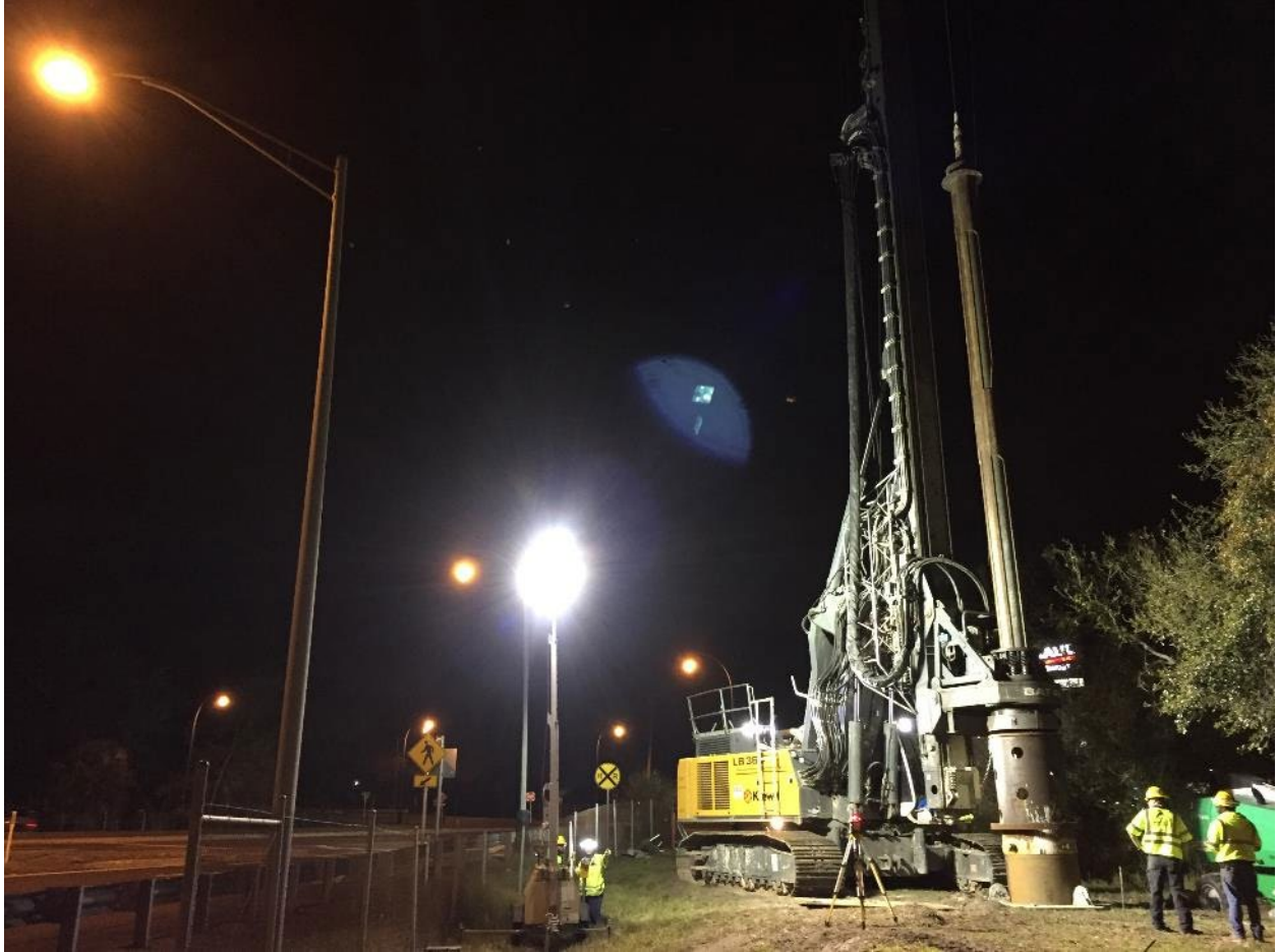
Figure 2-12. Drilling Test Shaft 4.
