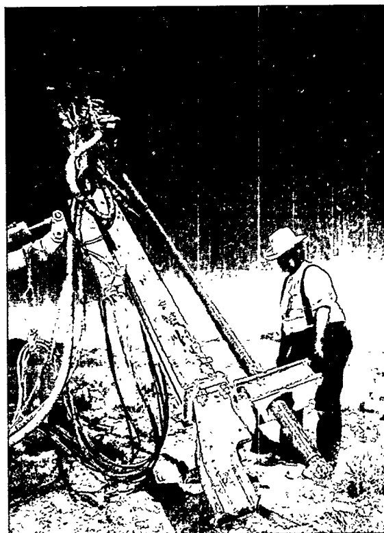
Constructing a monitoring station at Crater Flat
