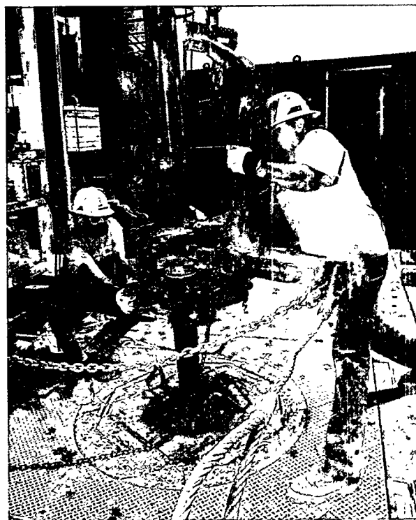
Drilling activities near Yucca Mountain
