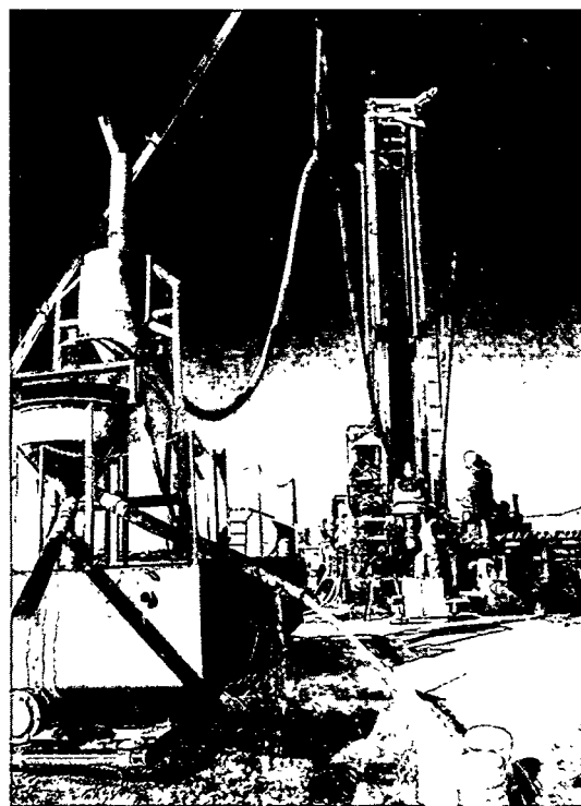
Nye County Early Warning Drilling Program
