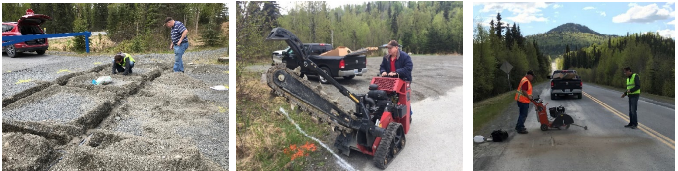
Figure 3 - Installation of Inductive Loops in Gravel and Asphalt Roadways
