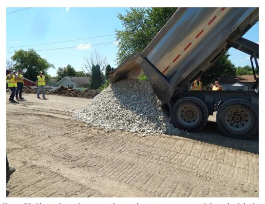
Figure 59. Photo. Dumping quarry by-product aggregate materials at the job site.
