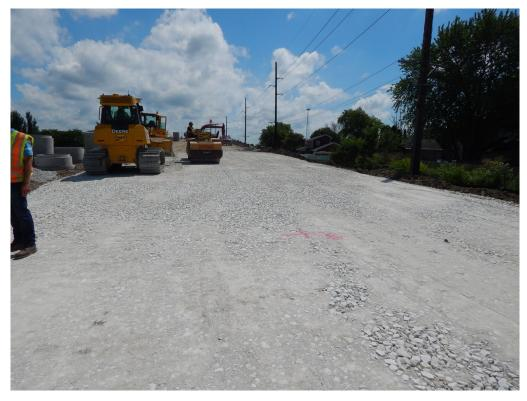
Figure 61. Photo. Final finished surface of the QBA\_M1 material after compaction.
