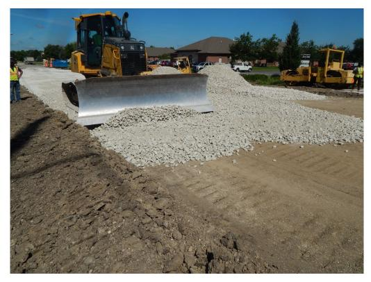
Figure 60. Photo. Spreading quarry by-product aggregate materials using a bulldozer.
