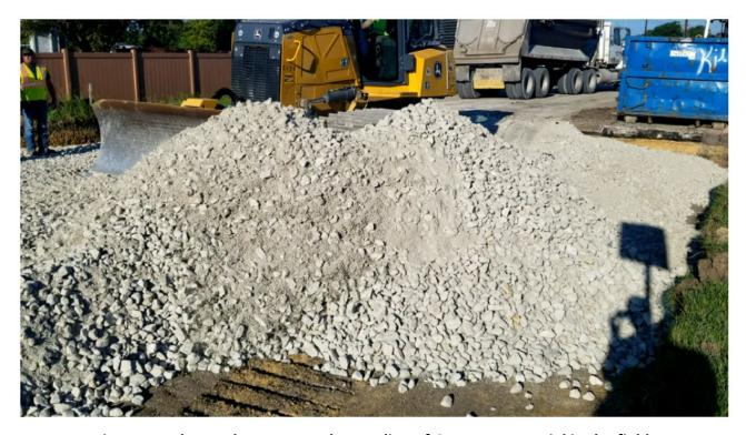
Figure 17. Photo. Placement and spreading of QBA\_M1 material in the field.
