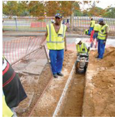
(b) Trenching for the conduit
