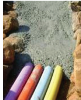
(c) Installed pipe with partial backfill
