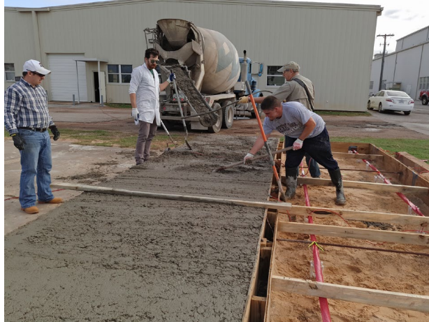
Figure 14a. Test slab placement.
