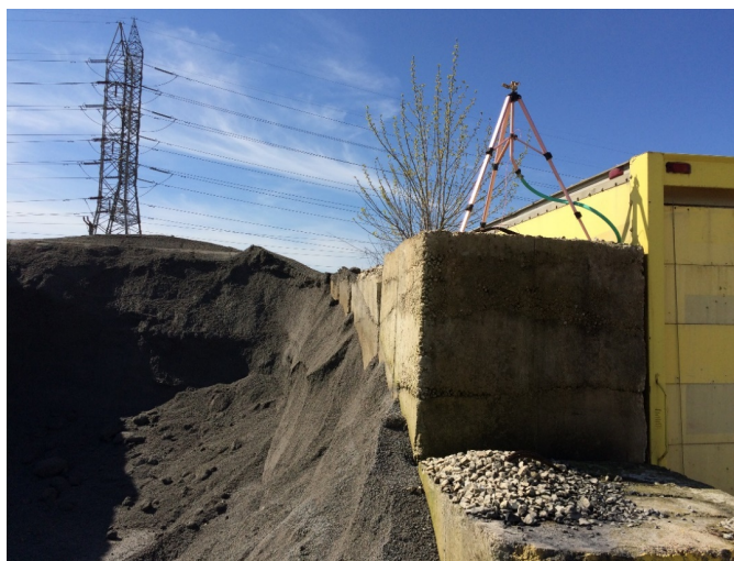
Figure 15. FLWA stockpile (Montanari et al. 2021).
