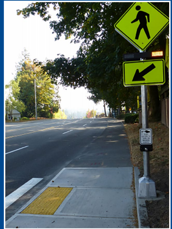
MaineDOT RRFB installation
