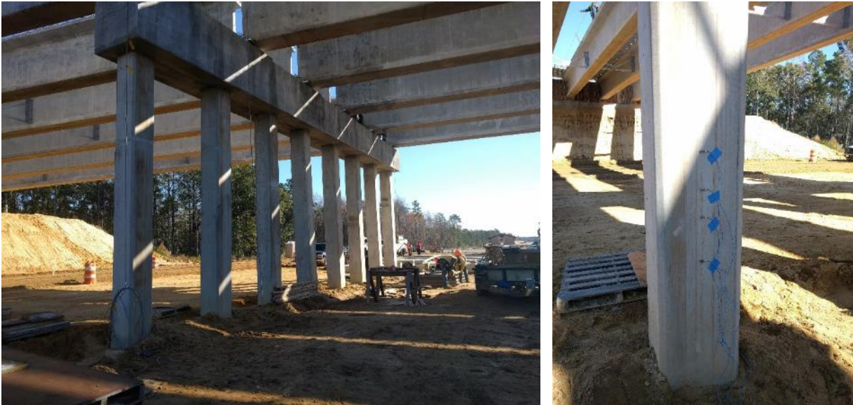
Figure 41: Wilmington, NC (a) Site (b) Instrumented piles
