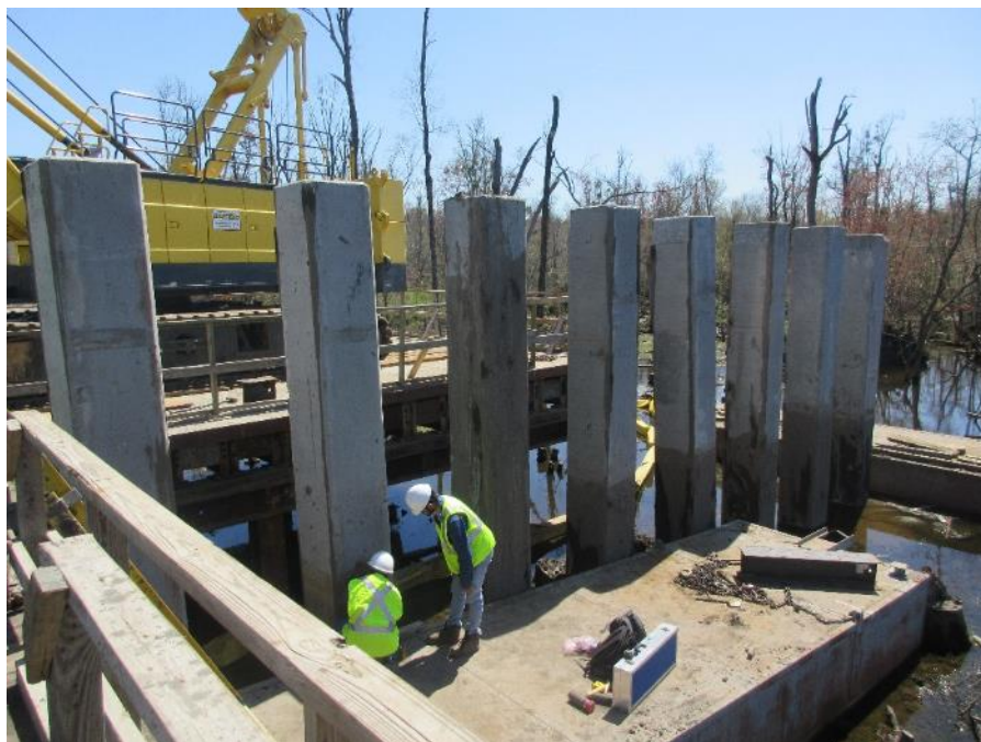
Figure 33: Kinston bridge site
