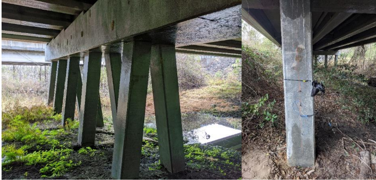
Figure 48: Wilmington 16 inch piles
