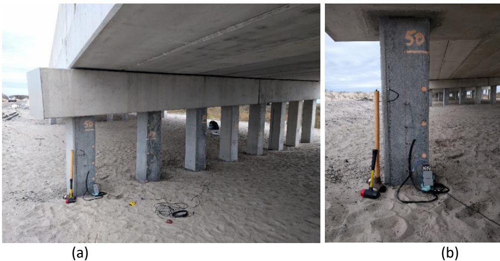
Figure 29: Rodanthe piles with pile cap (a) site (b) instrumented pile
