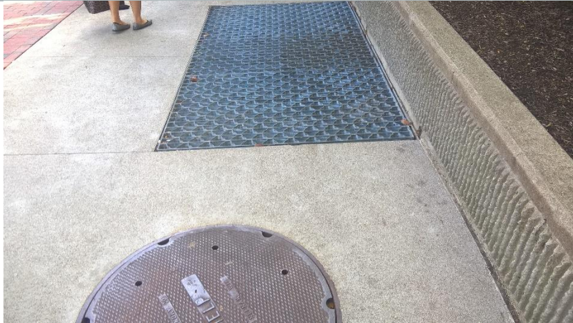
This picture shows a grate in the sidewalk.
