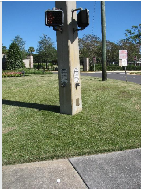
This is a bad example of an out of reach pedestrian pushbuttons.
