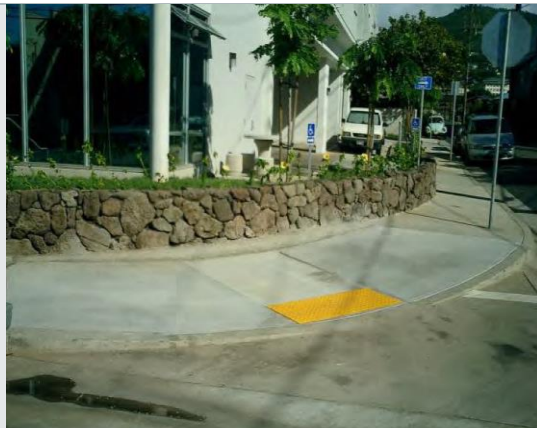
This is an example of a good parallel ramp.
