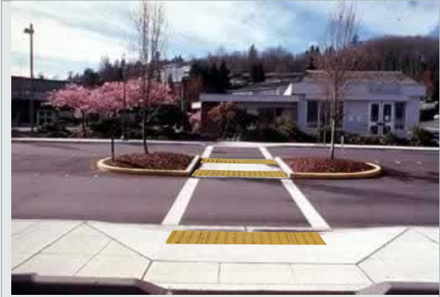
This is a good example of a median cut-through.
