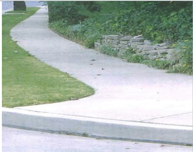
This picture shows a missing curb ramp.
