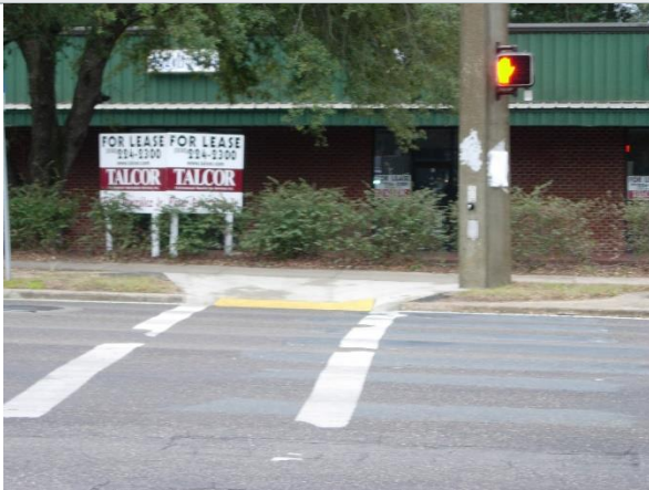
This picture shows a curb ramp in good condition.
