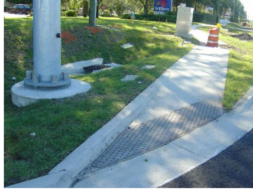
This is an example of a good linear ramp.
