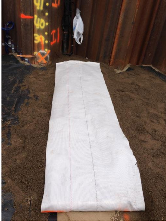
Figure 22. Fiber optic strain gauge field installation
